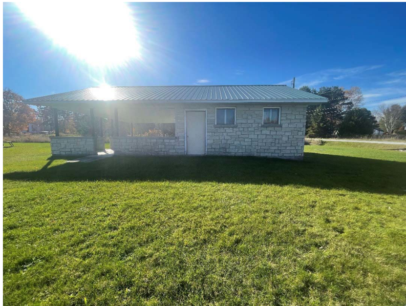
Photo 1 – Exterior of Pavilion. Entrance door 1 to pavilion.
