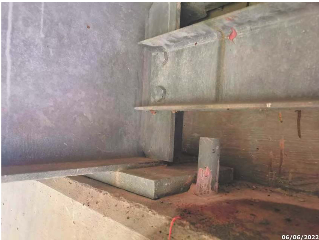
South abutment typical bearing
