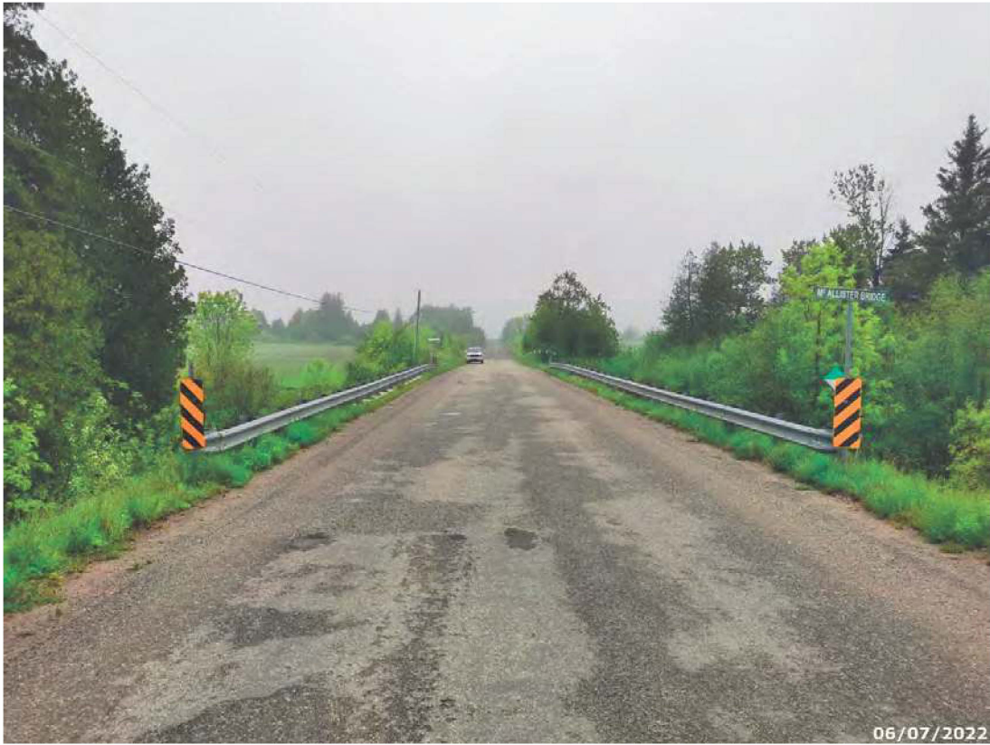
Looking North Across The Structure
