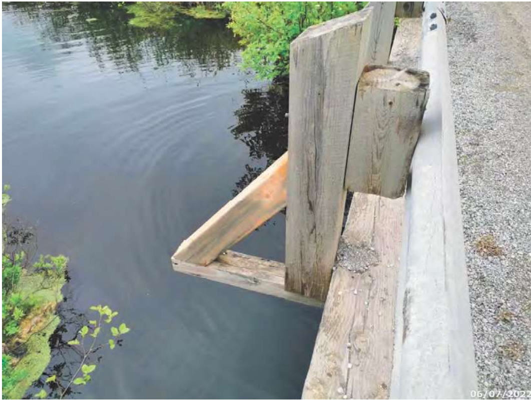
Typical railing posts and supports
