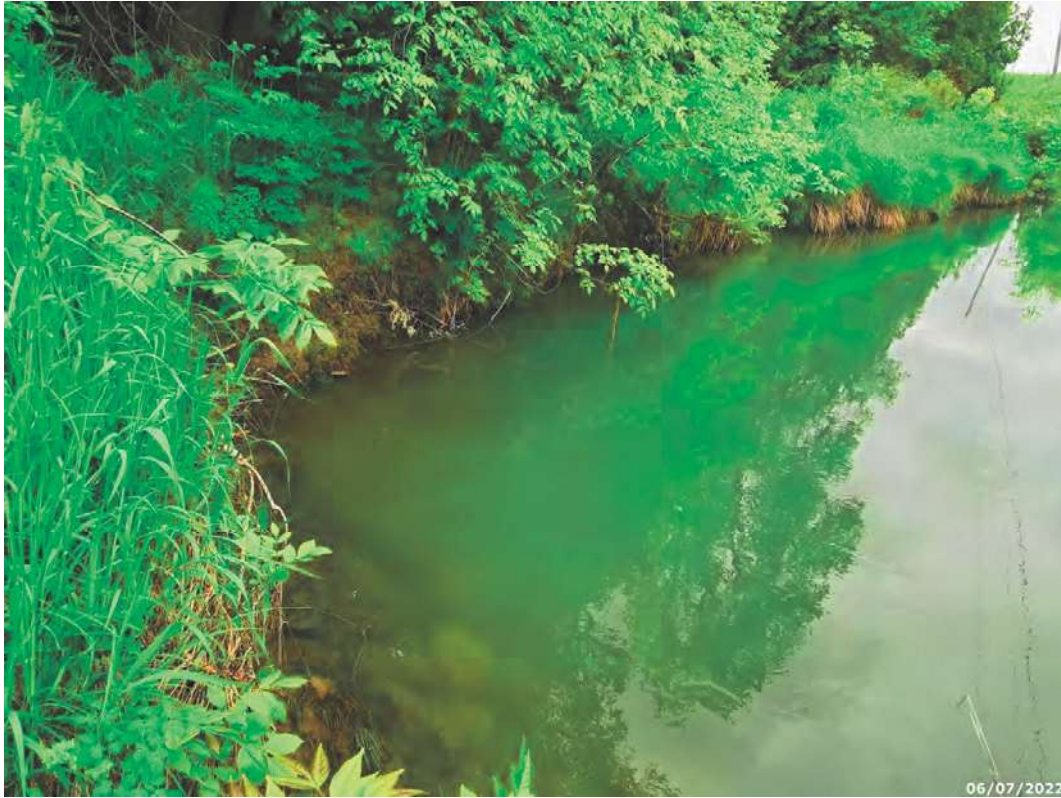
Upstream scour and undermining
