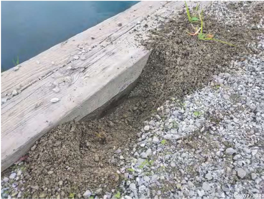
Plugged scupper drain in curb
