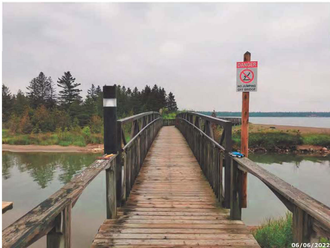
Looking south across structure
