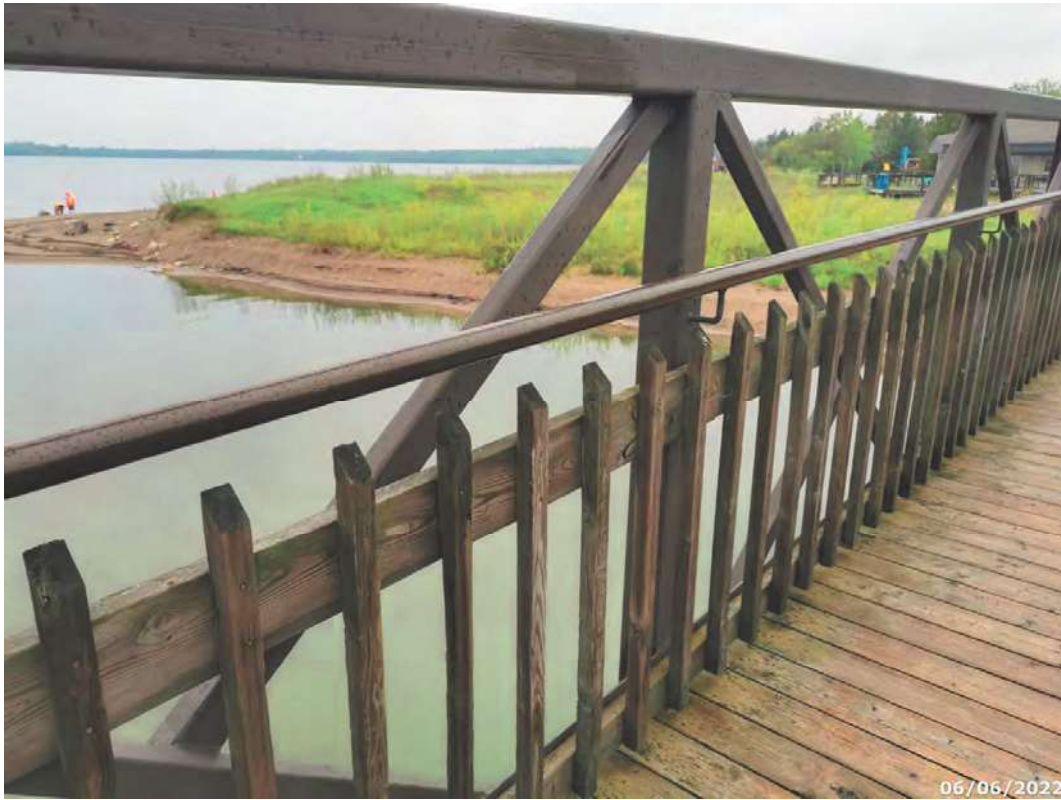
Typical hand railing arrangement
