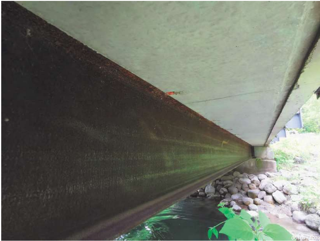
Typical exterior soffit
