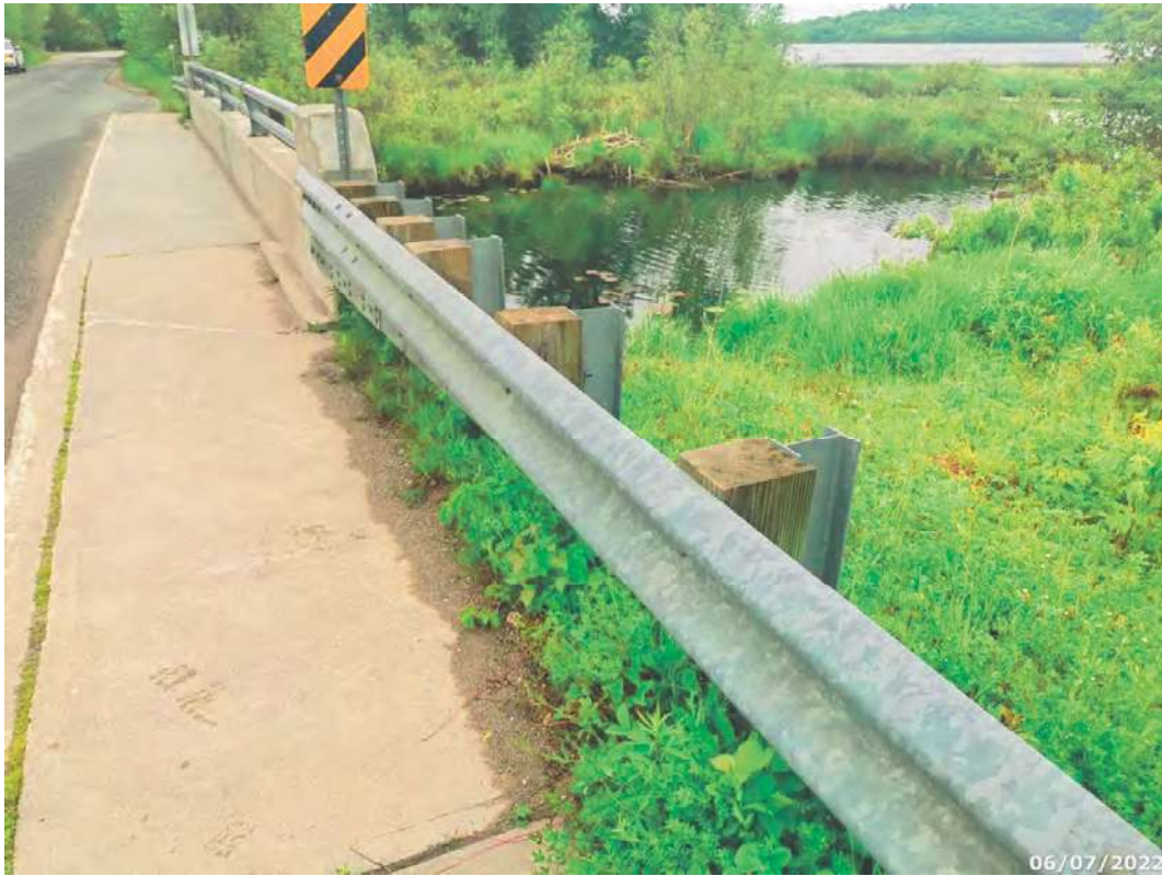
Typical approach guiderail
