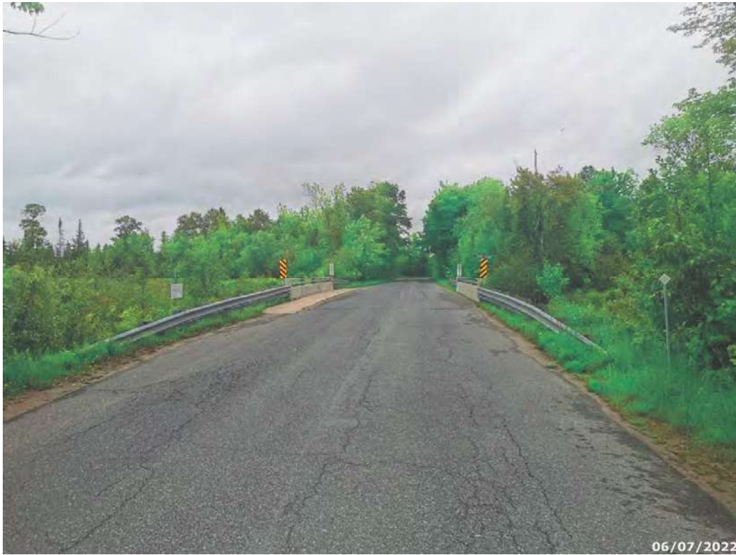
Looking east across structure
