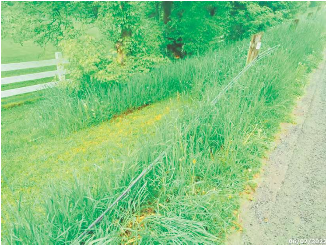
Broken and missing guiderail post in northwest quadrant
