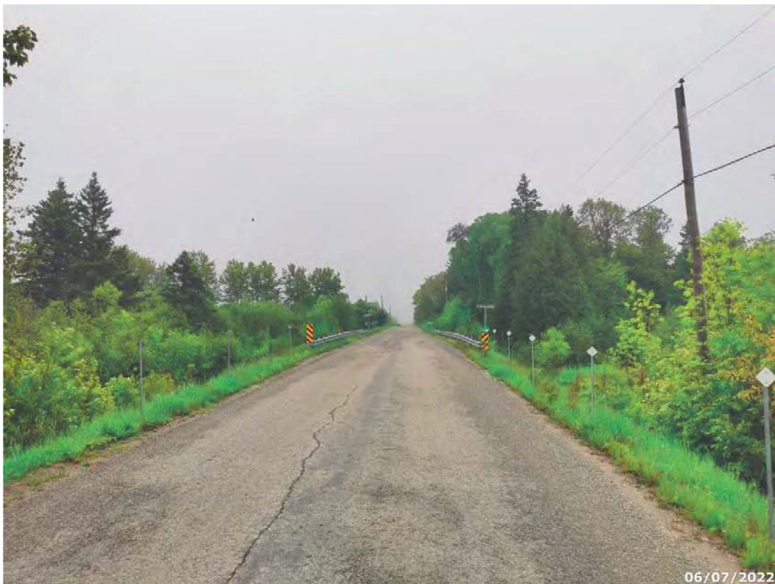
Looking South Across The Structure
