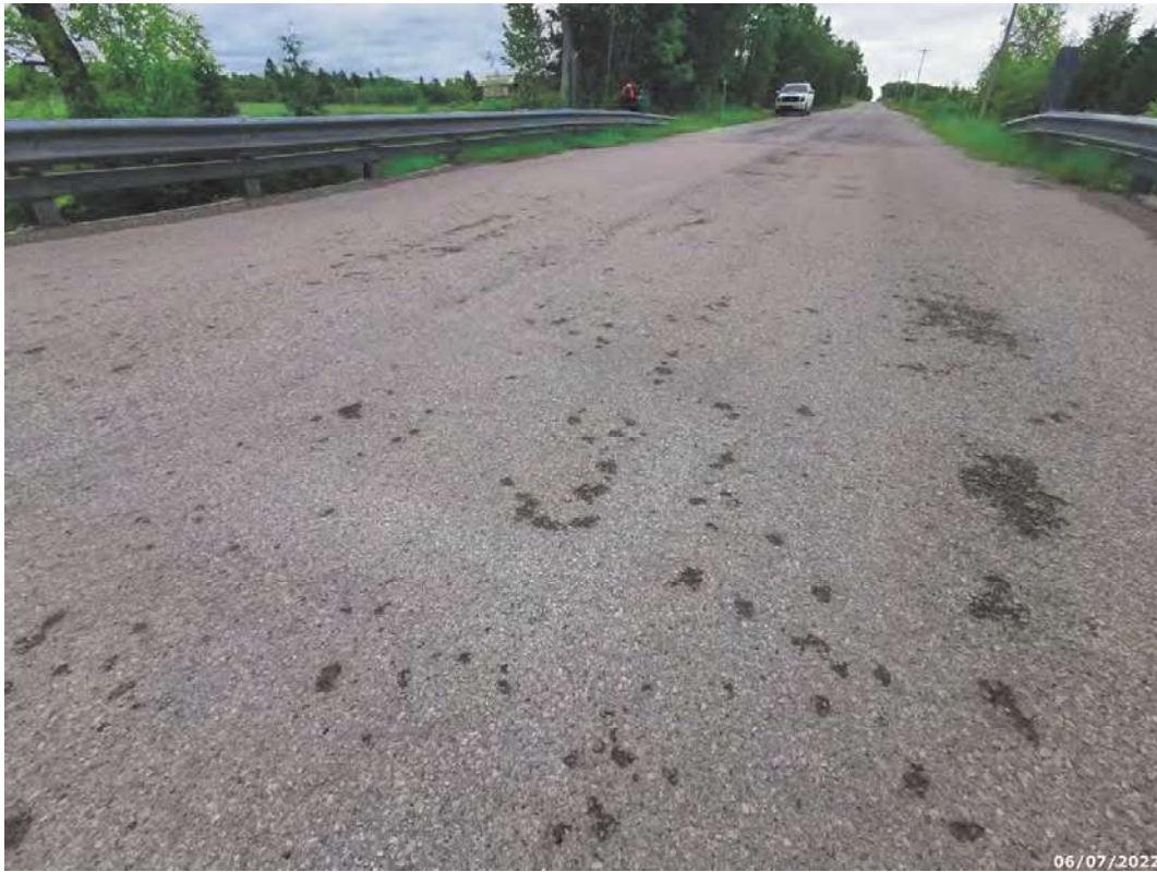
Typical deck wearing surface
