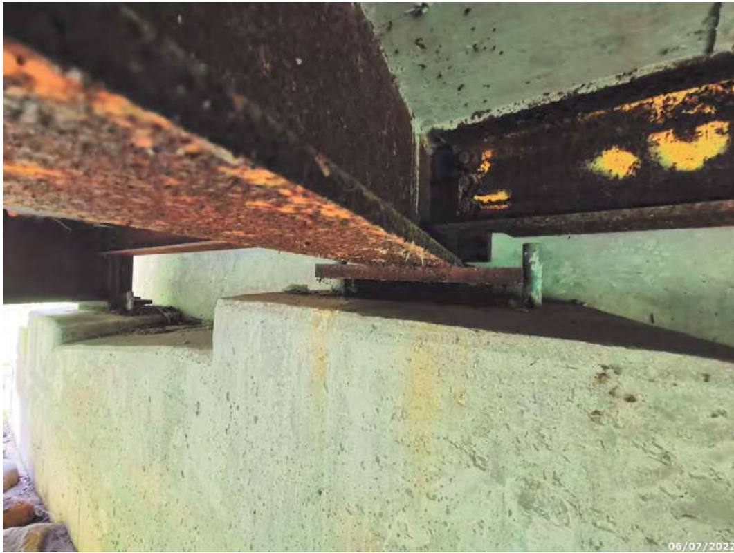
Center girder bearing, west abutment
