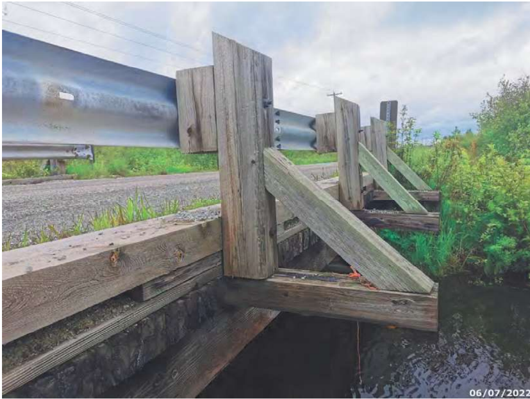
Typical railing support
