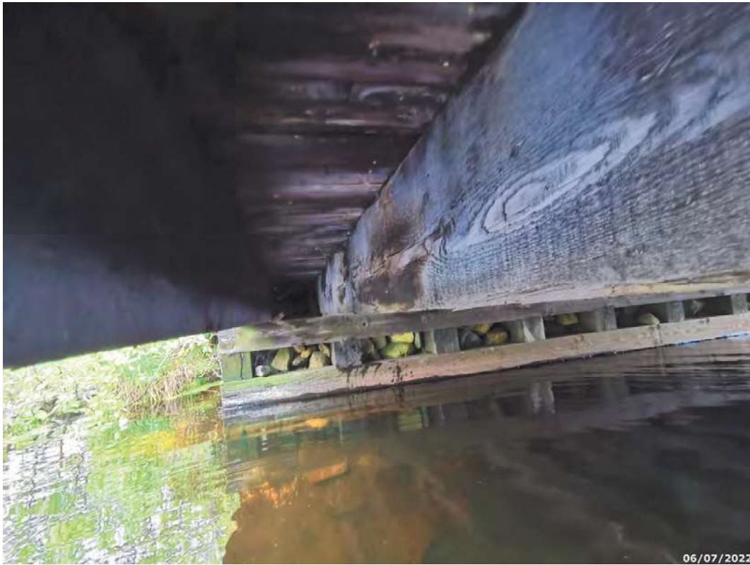
Typical exterior soffit
