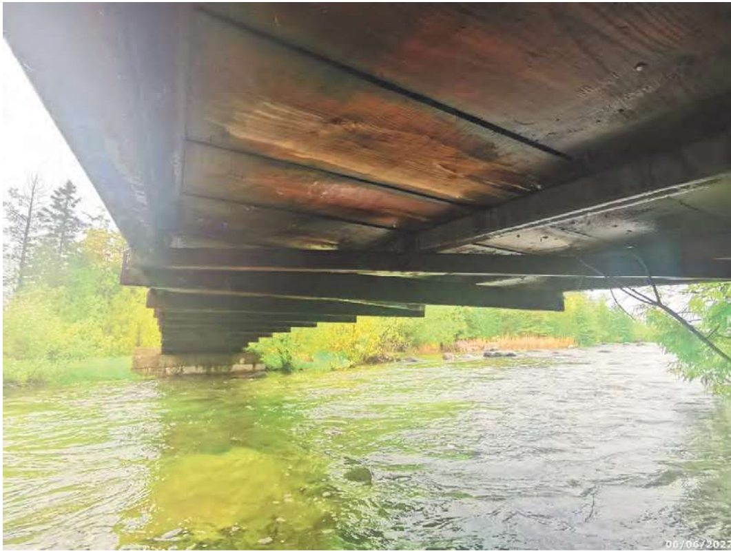
Deck soffit looking north
