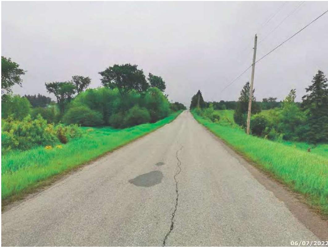
Looking east across structure
