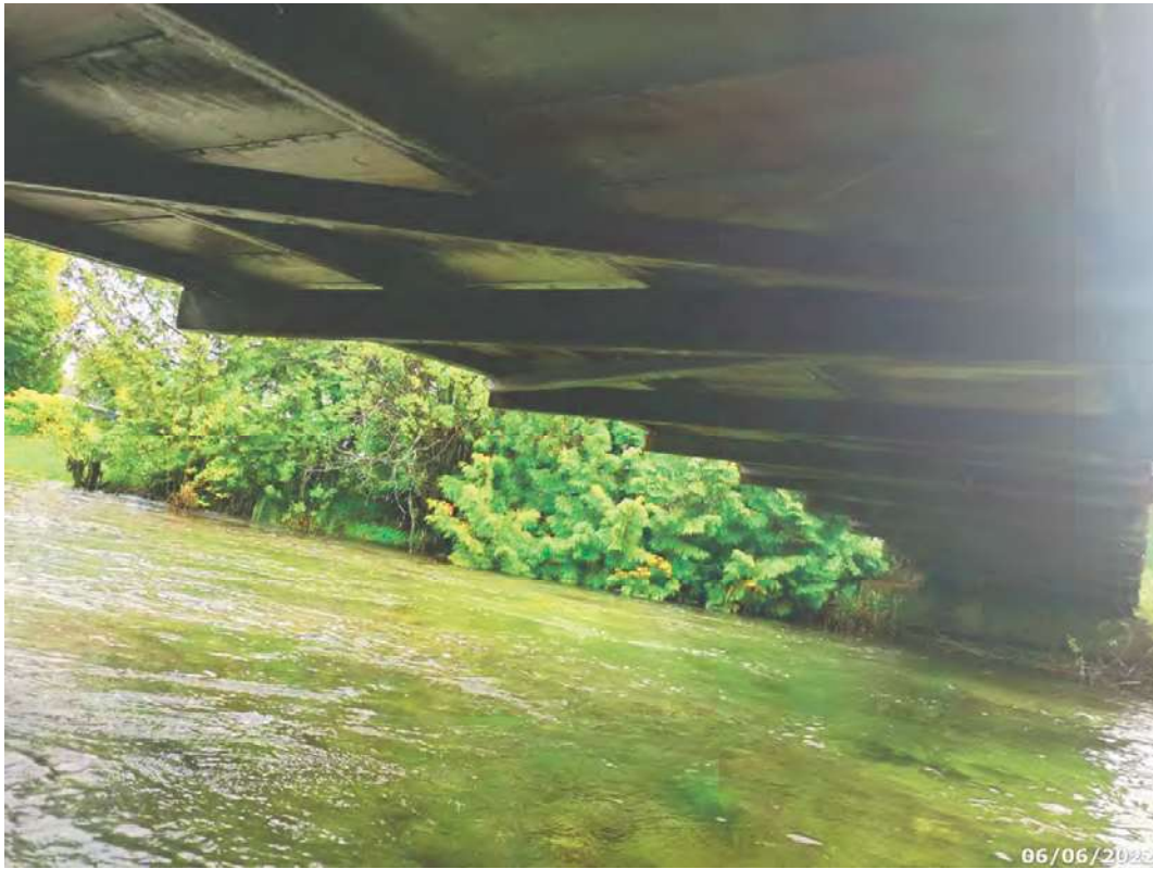
Typical deck soffit looking south
