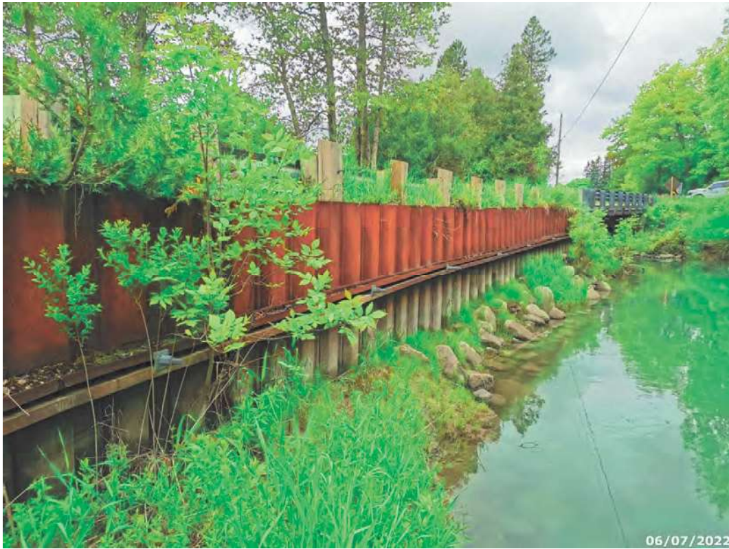
Sheet pile general arrangement, northeast embankment
