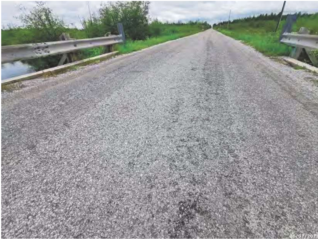
Typical deck wearing surface
