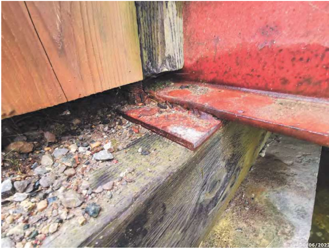
Typical bearing plate at east abutment (exterior beams only)
