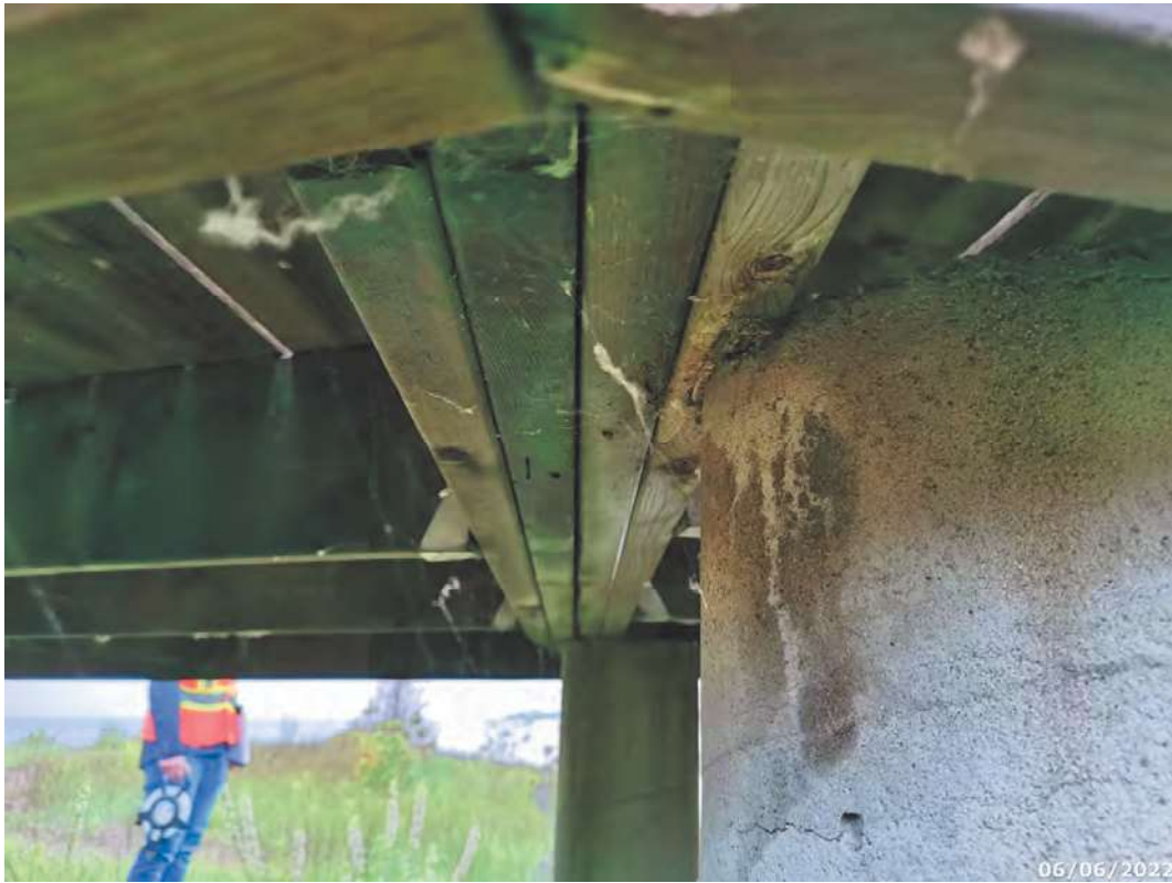
Minimal approach sidewalk bearing
