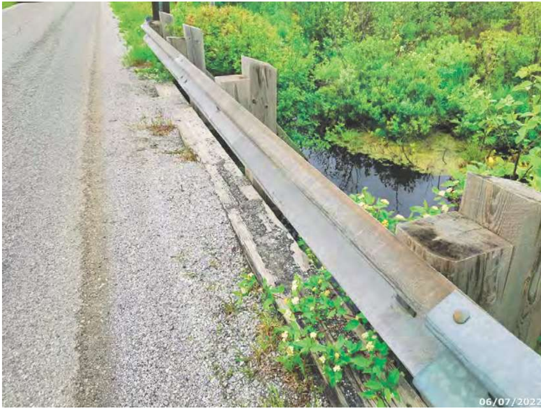
Typical Barrier system
