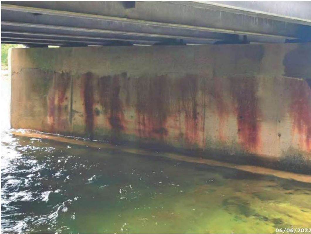
Pier arrangement looking south
