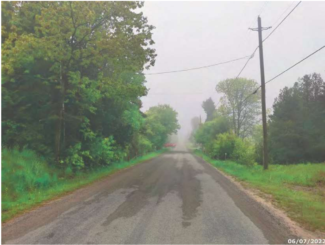
Looking west across structure
