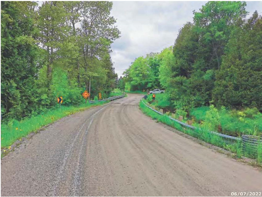
Looking West Across The Structure
