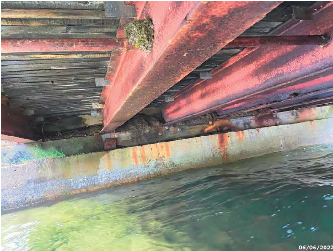
Typical end soffit
