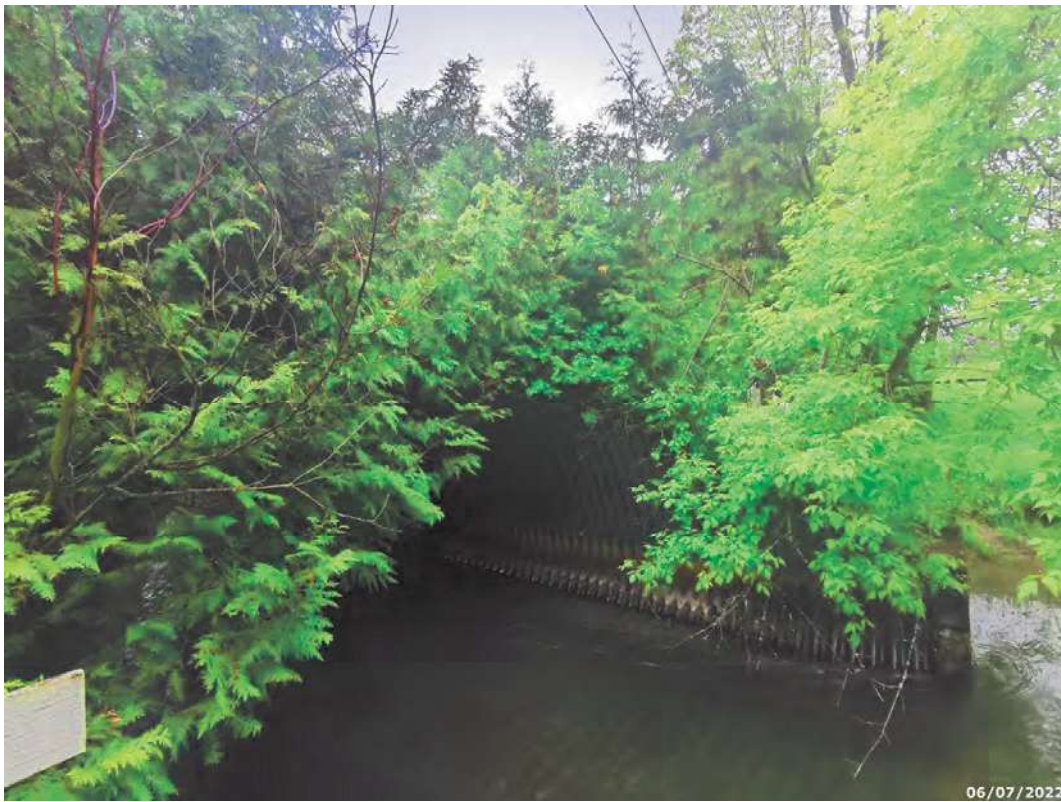
Severe tree growth around inlet components
