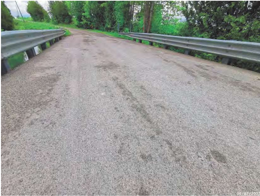
Typical deck wearing surface
