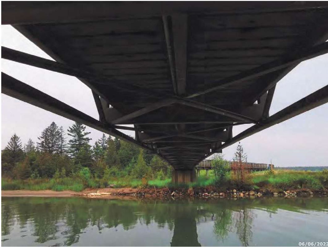
Deck soffit general arrangement, looking south
