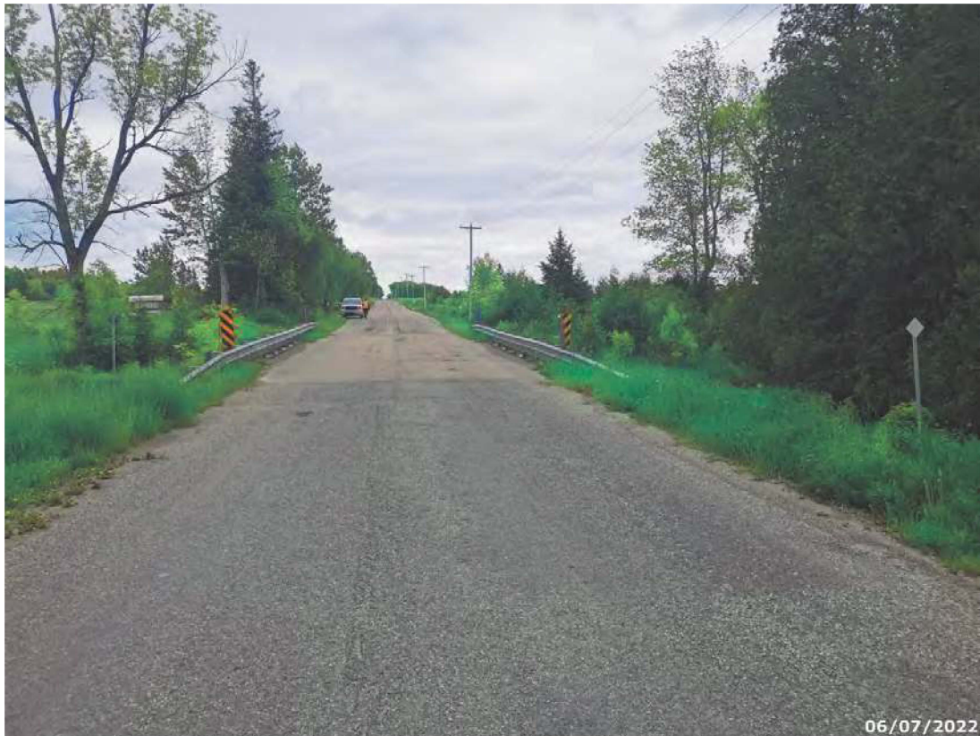
Looking south across structure
