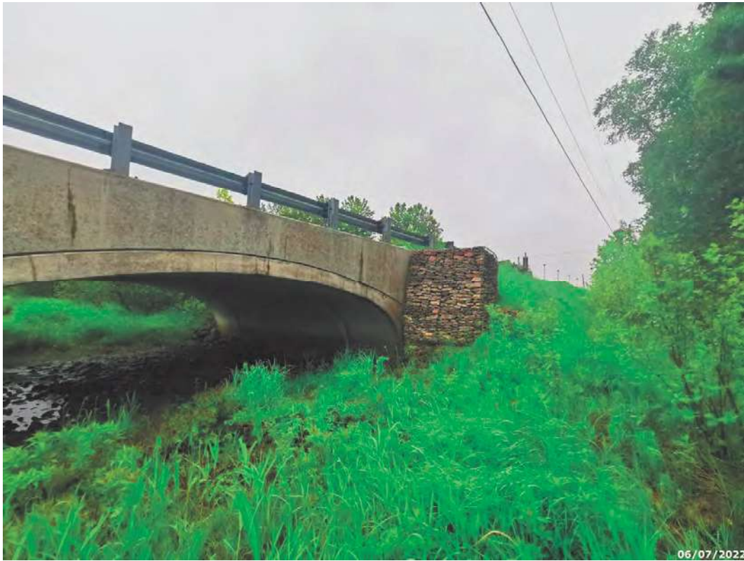
Southwest gabion basket embankment
