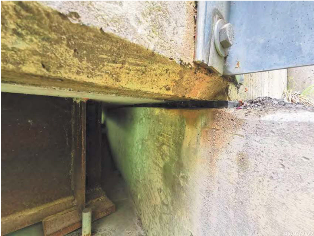
Neoprene bearing pad along deck over ballast wall joint
