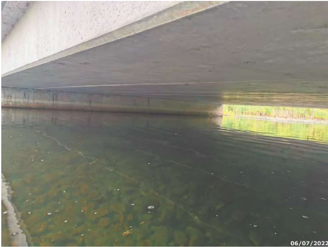
Typical west abutment general arrangement
