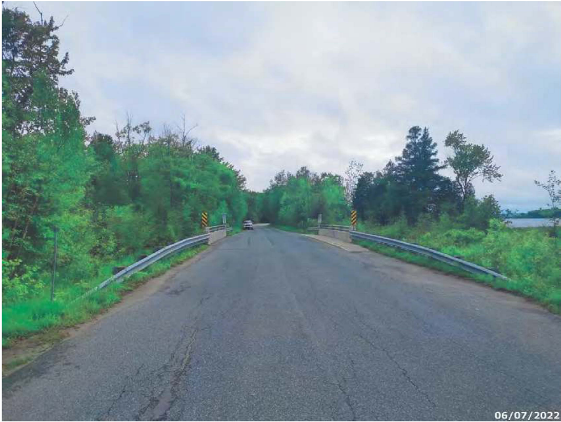
Looking west across structure
