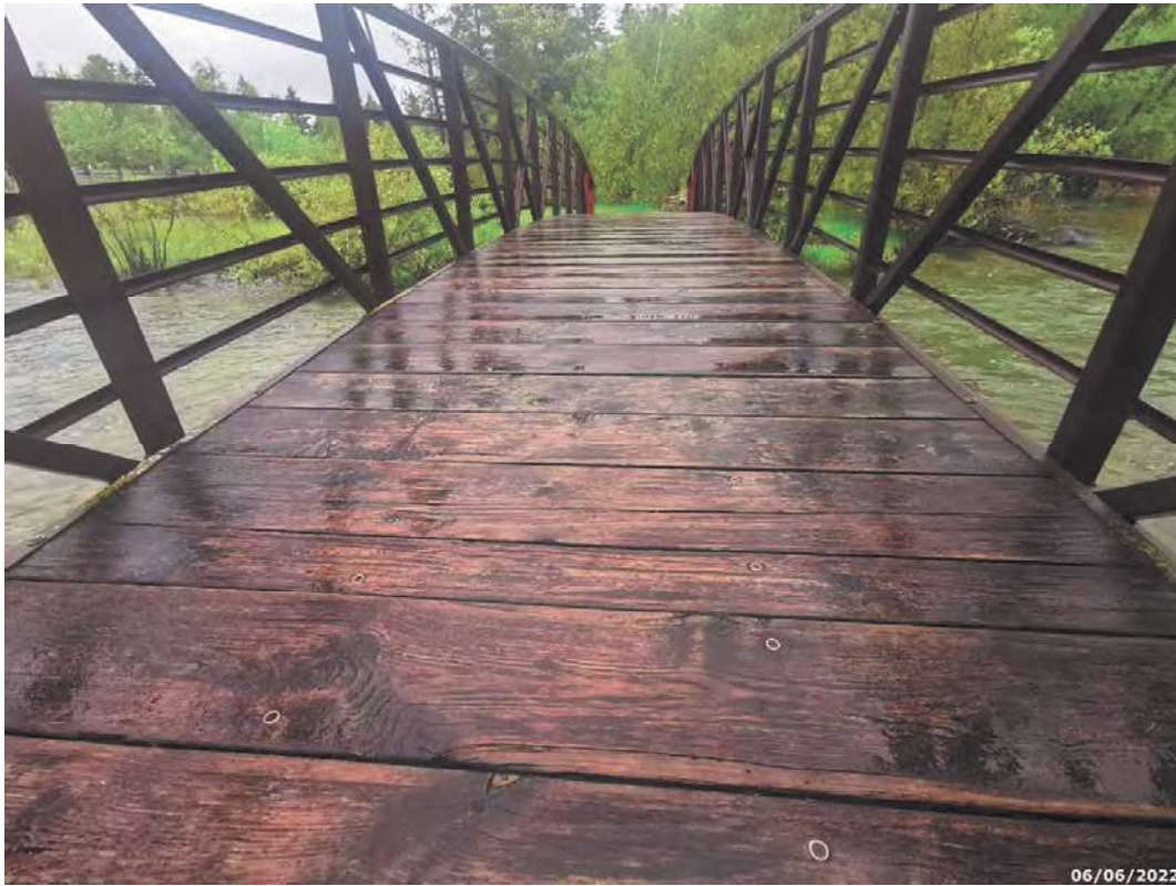
Typical deck wearing surface
