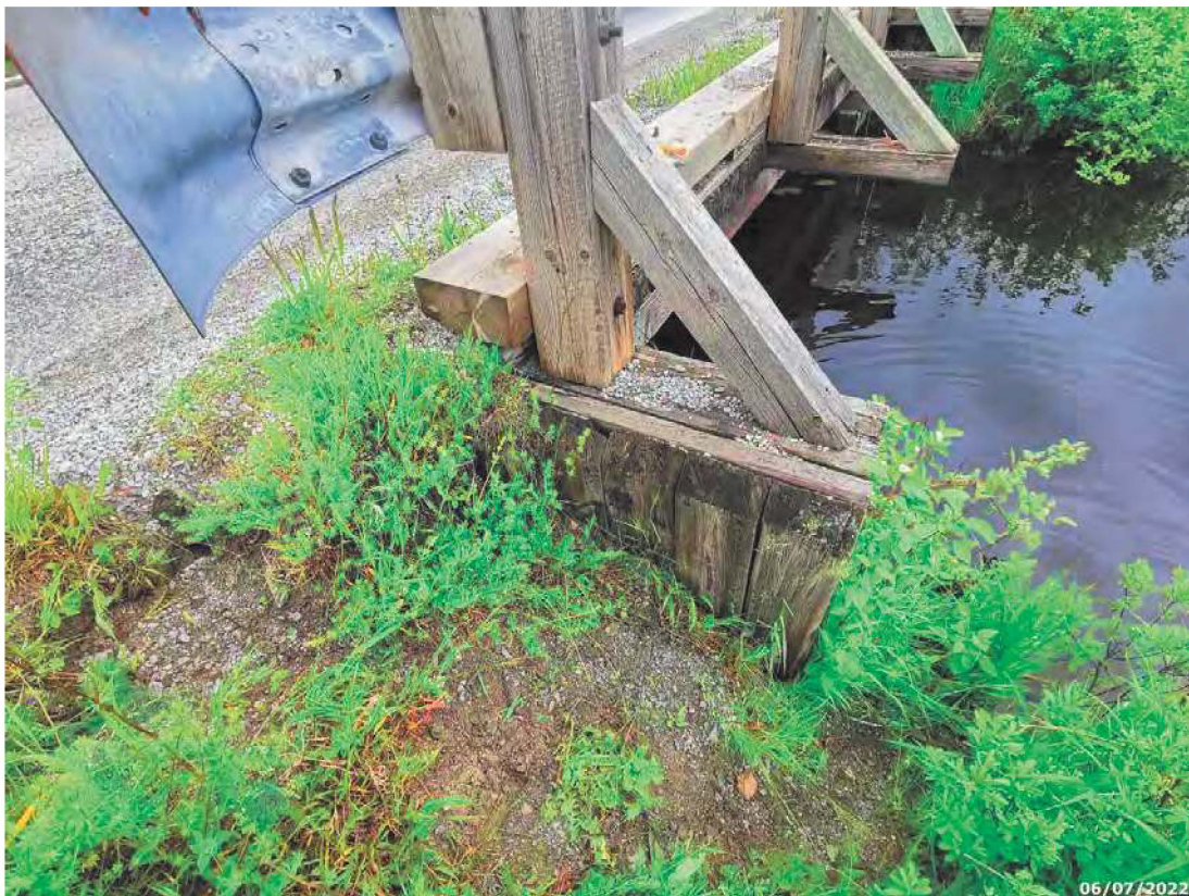
Exposed ballast wall, southwest quadrant
