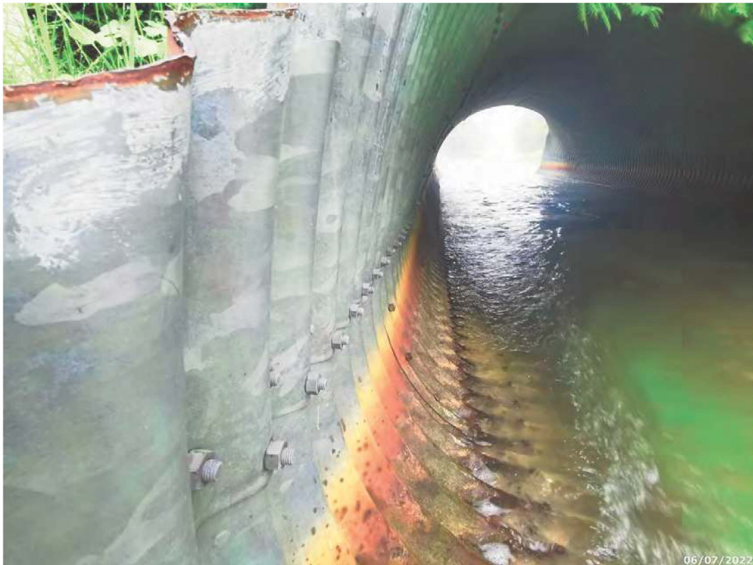
Looking south through culvert barrel, along east wall
