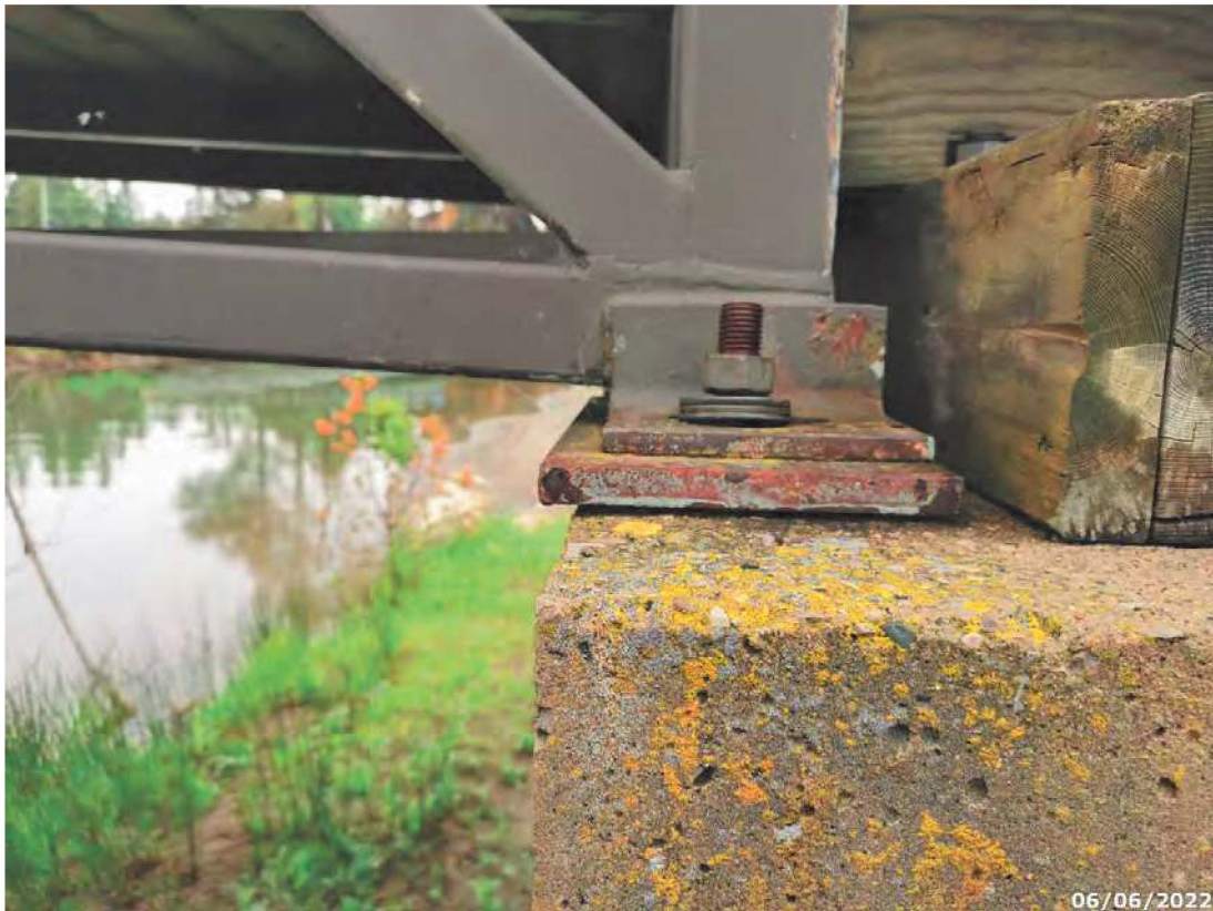
South bearing general arrangement, loose anchor nuts
