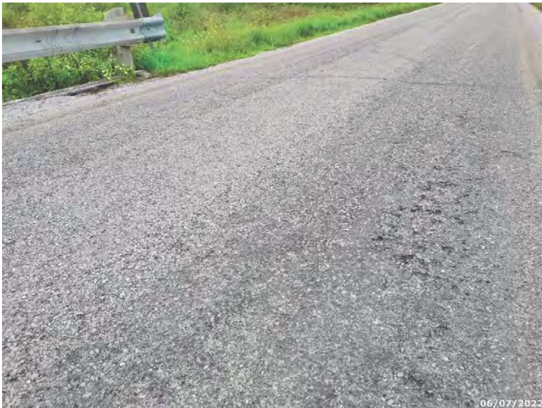
Typical deck wearing surface with localized moderate ravelling and light rutting
