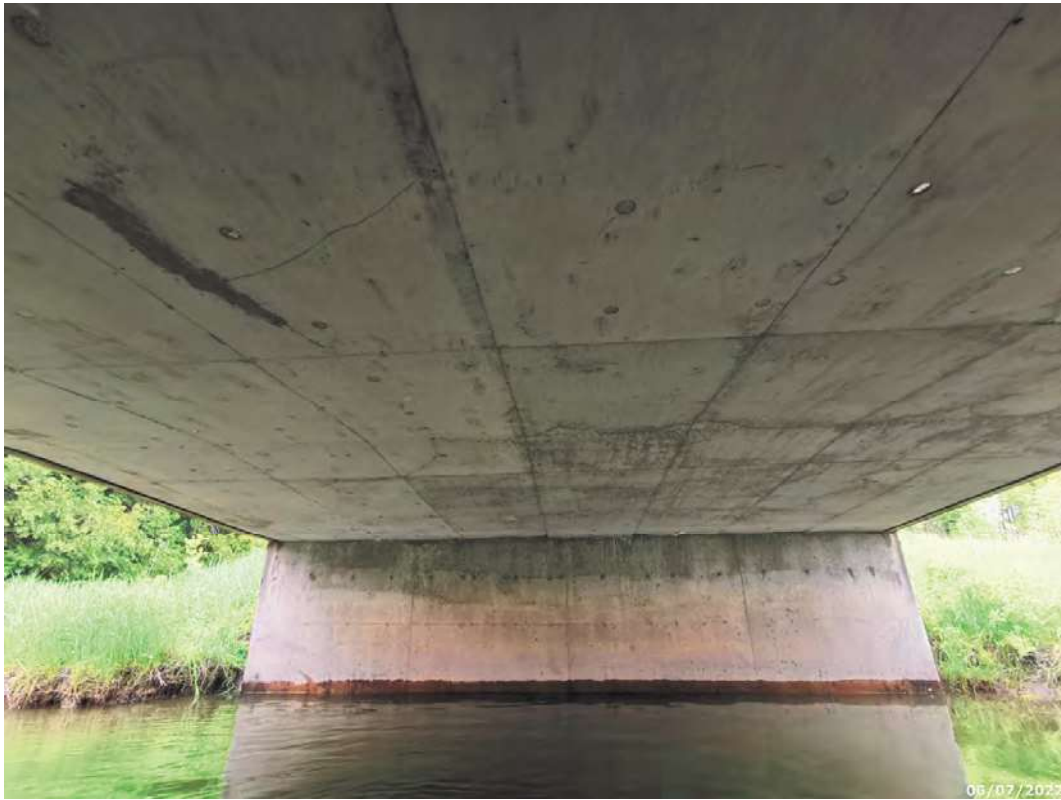
Soffit general arrangement, looking north
