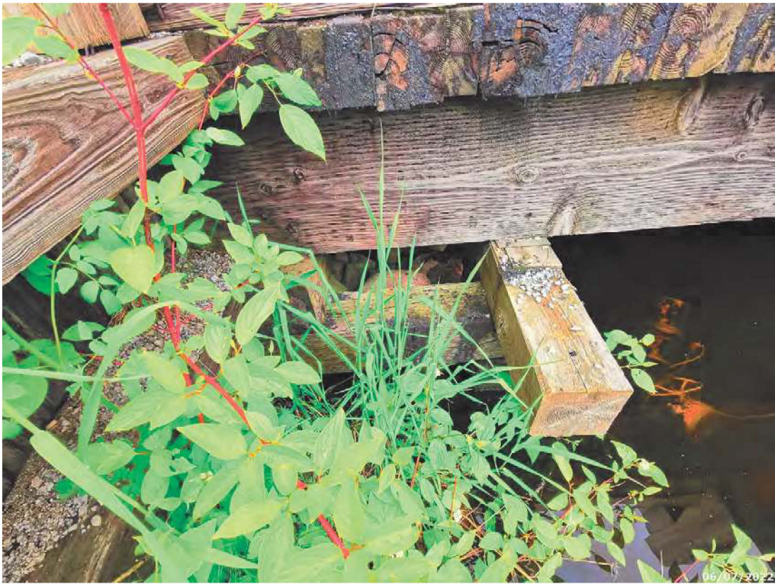
Typical abutment crib
