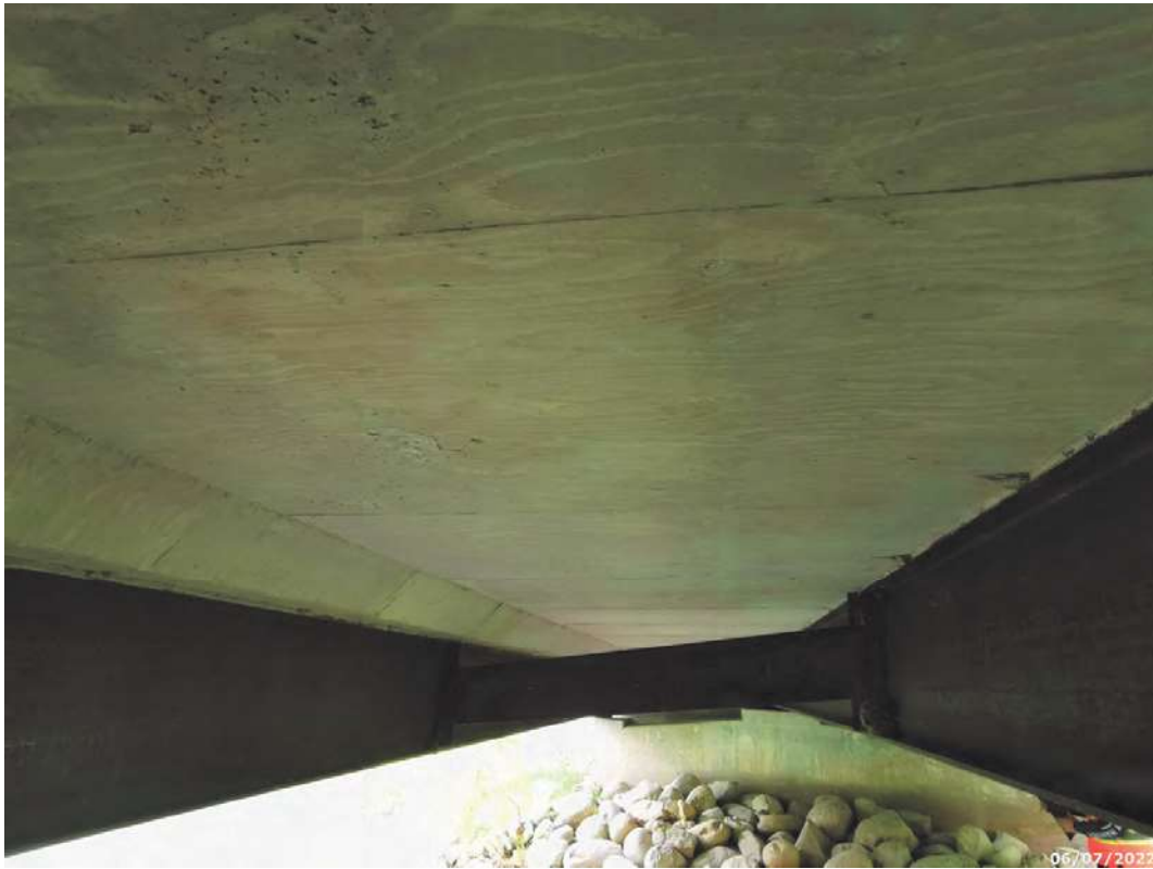
Typical interior soffit
