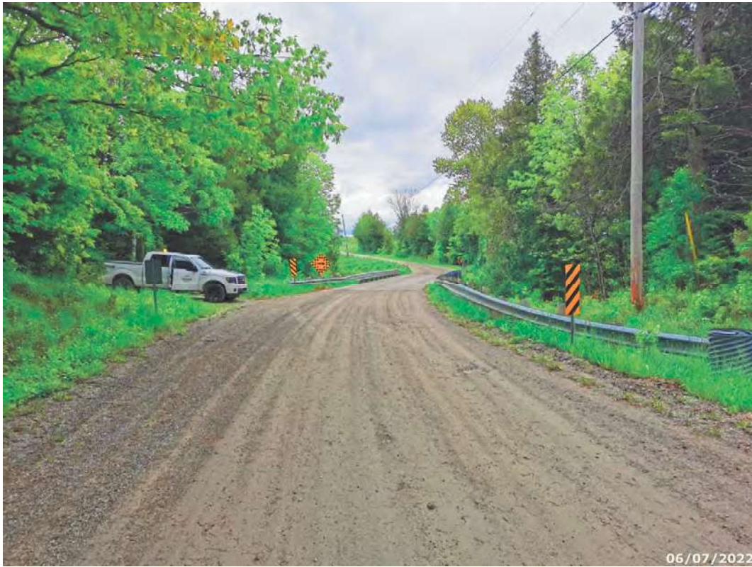
Looking east across structure
