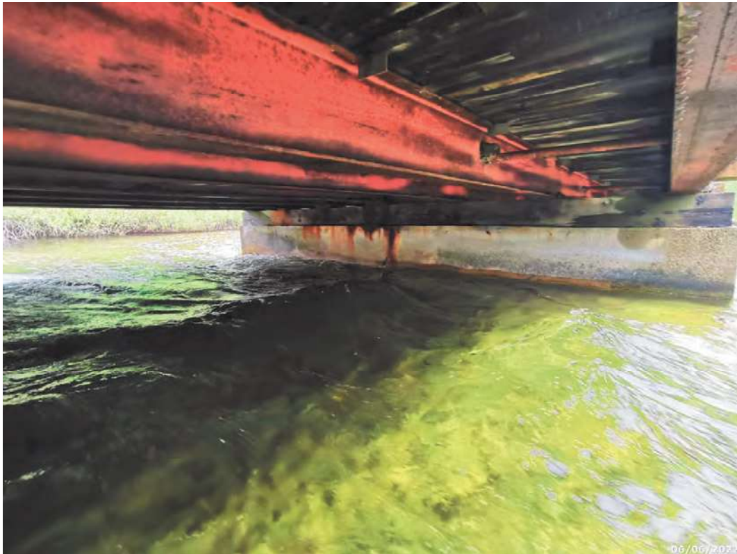
Typical exterior soffit
