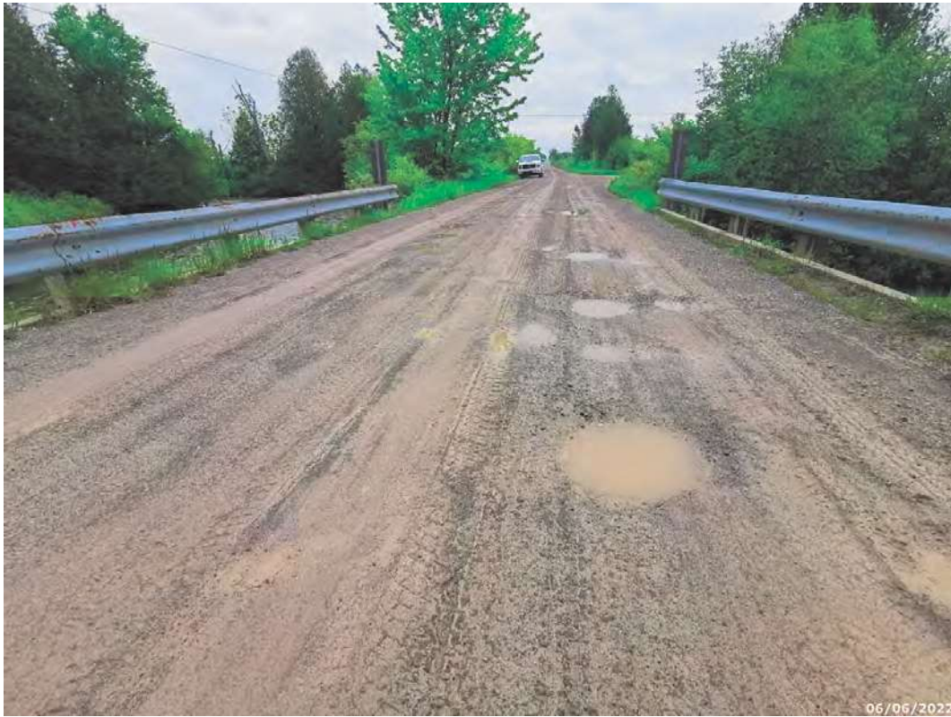
Typical Deck Wearing Surface
