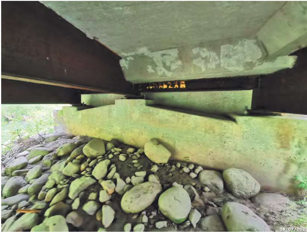
East abutment general arrangement
