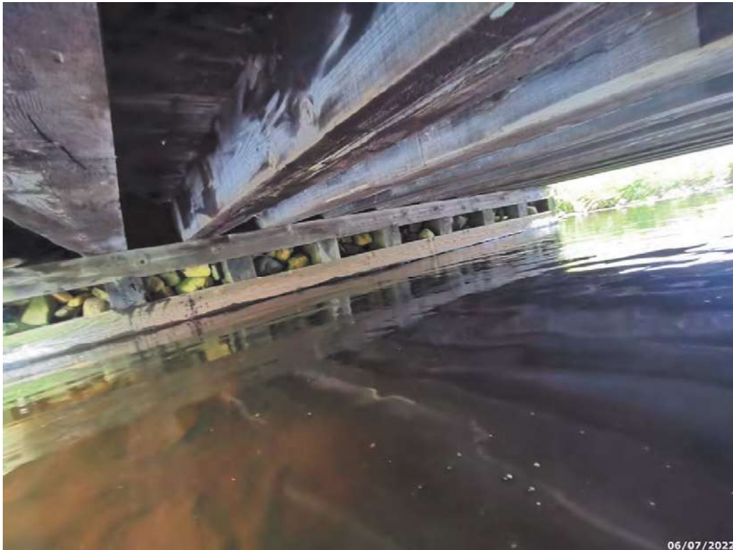
Typical stringer general arrangement
