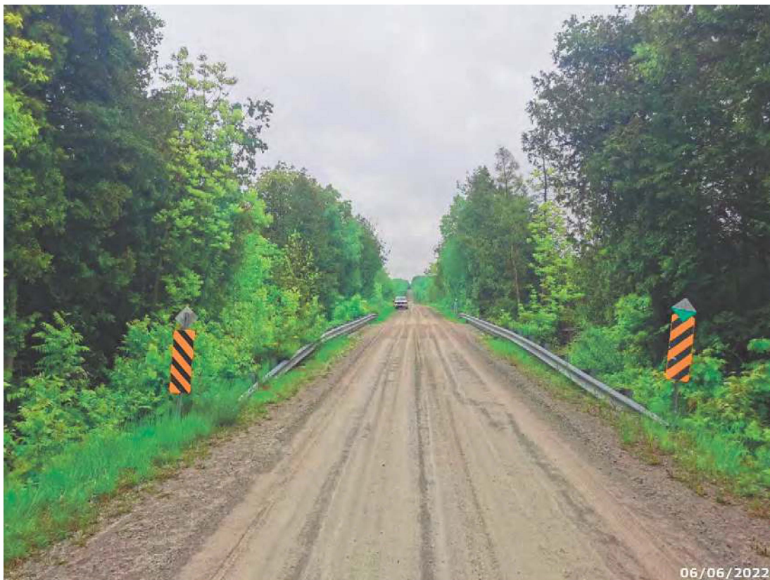
Looking south across structure
