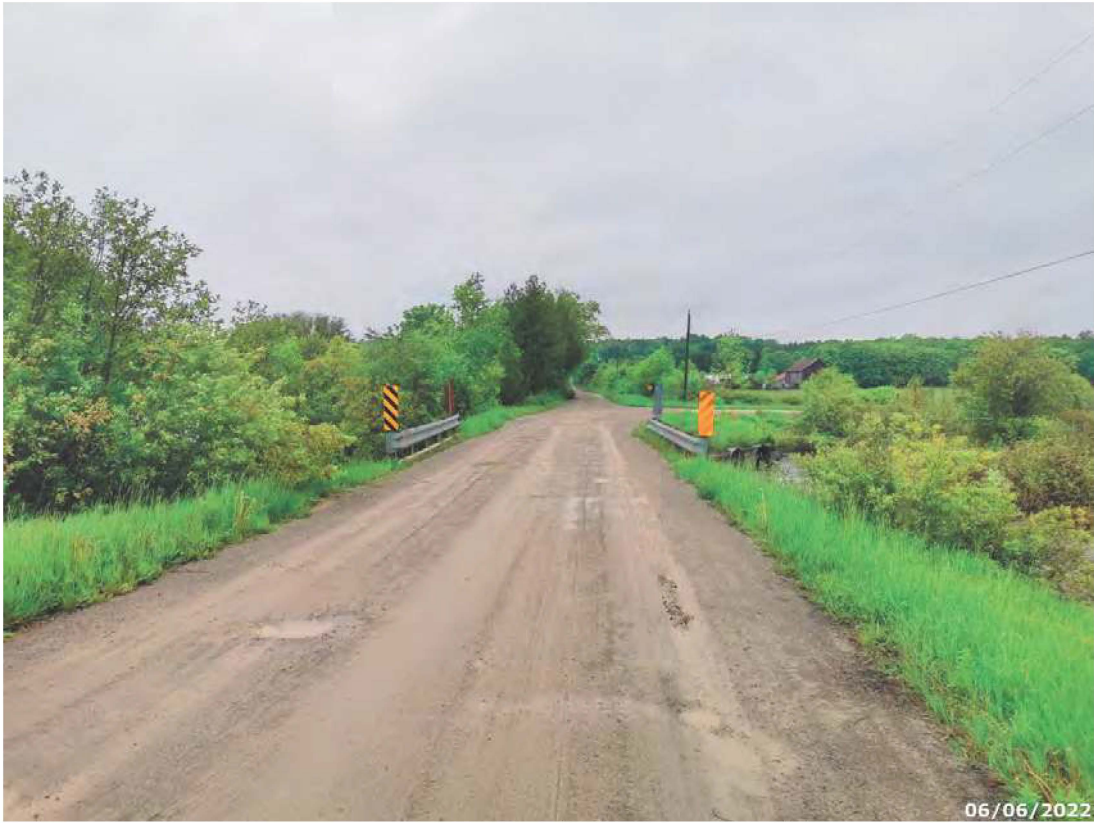
Looking West Across The Structure
