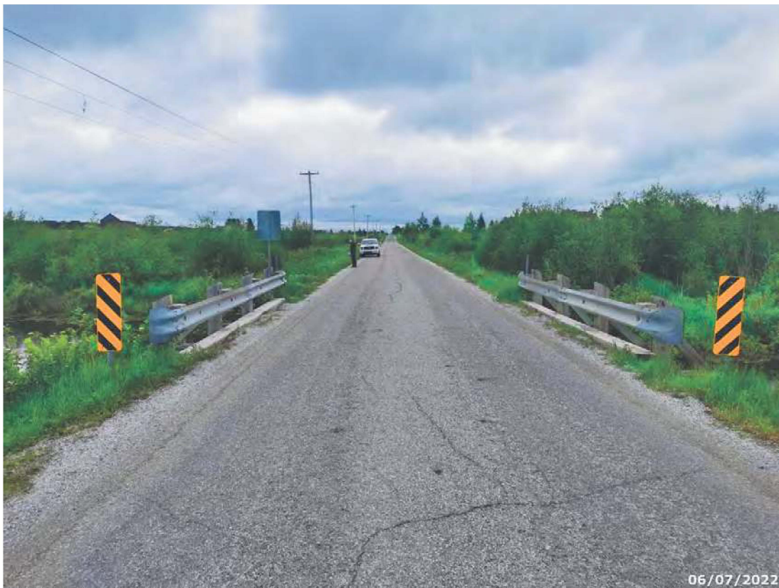
Looking east across structure
