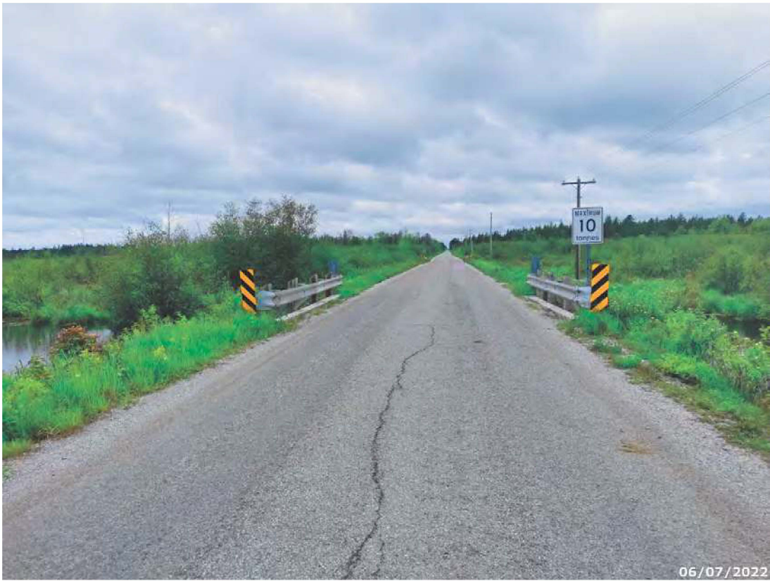
Looking west across structure
