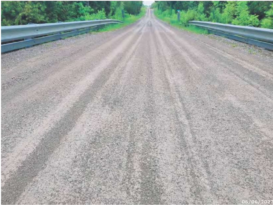
Typical deck wearing surface
