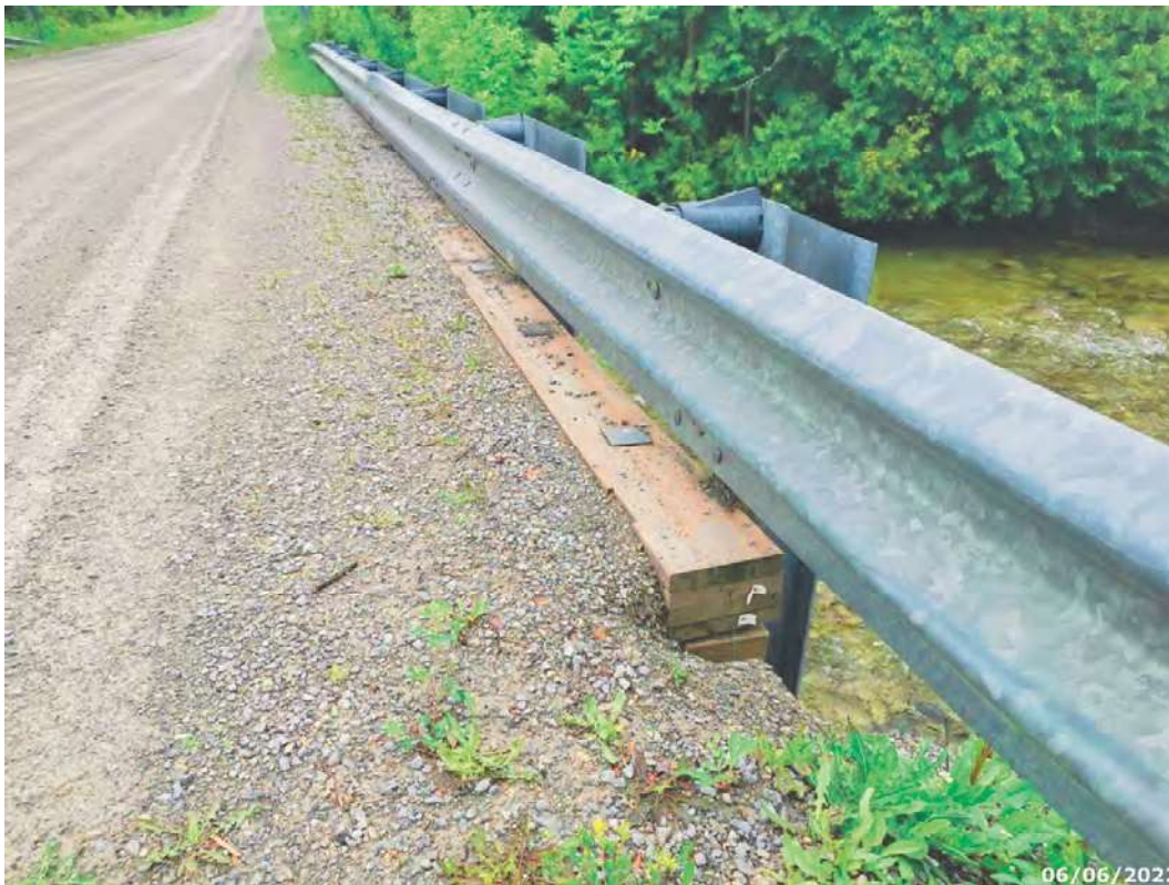
Typical guiderail system, buried curb, minor erosion channel at southwest corner
