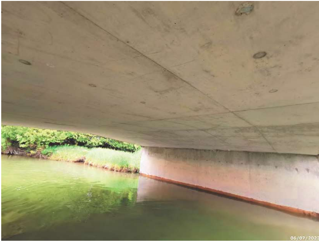
Soffit general arrangement, looking south
