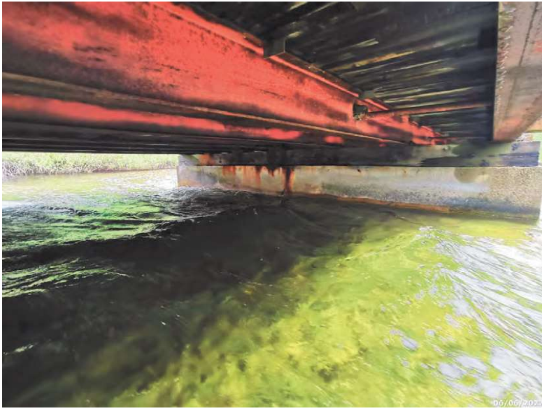
Pier general arrangement, looking east
