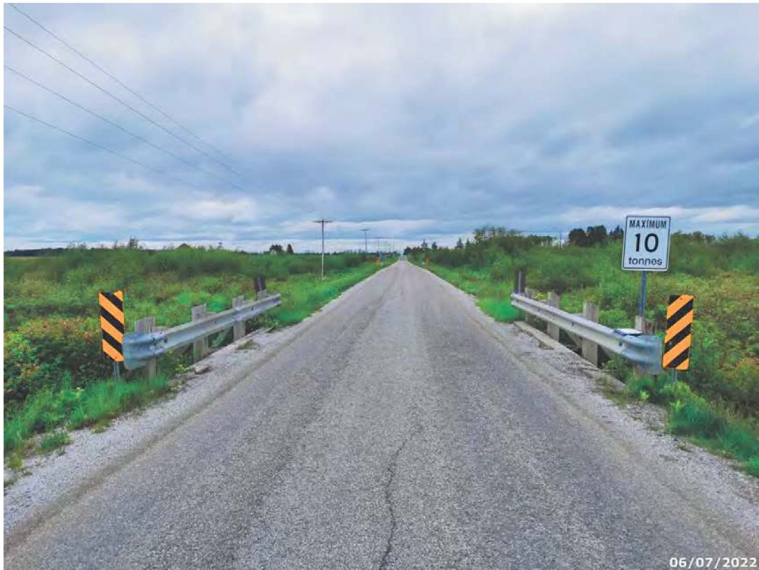
Looking east across structure
