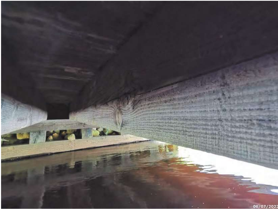
Typical interior soffit
