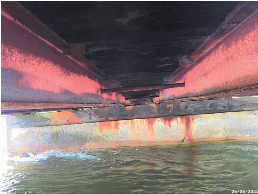
Typical interior soffit
