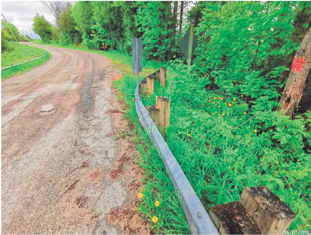
Southeast guiderail (typical)
