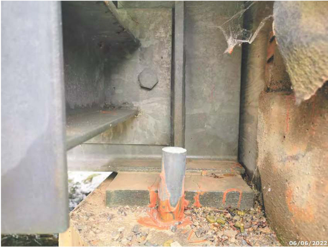
South abutment typical bearing
