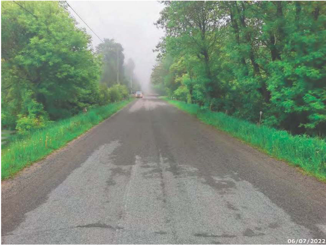
Looking East Across Structure
