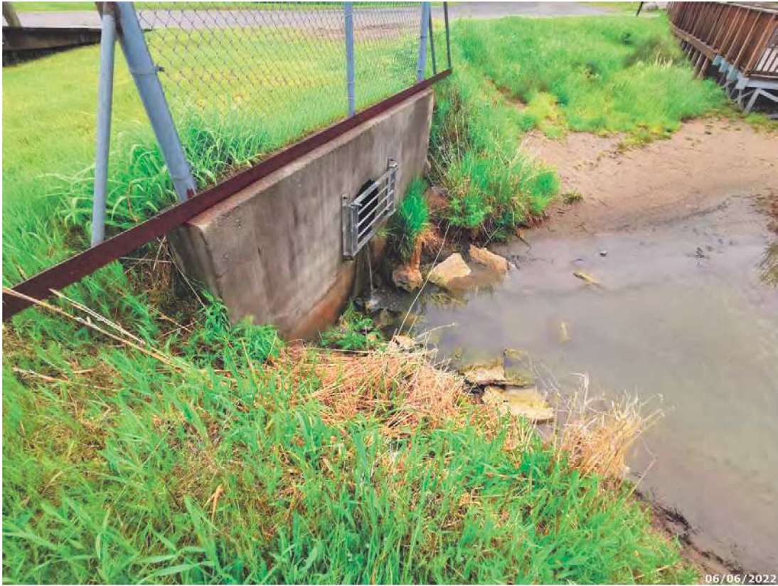
Storm sewer outlet, northeast of bridge
