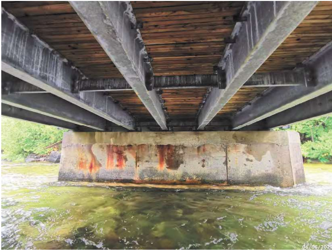
Interior soffit looking north
