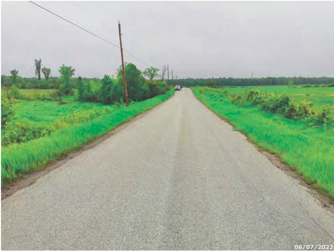
Looking West Across The Structure
