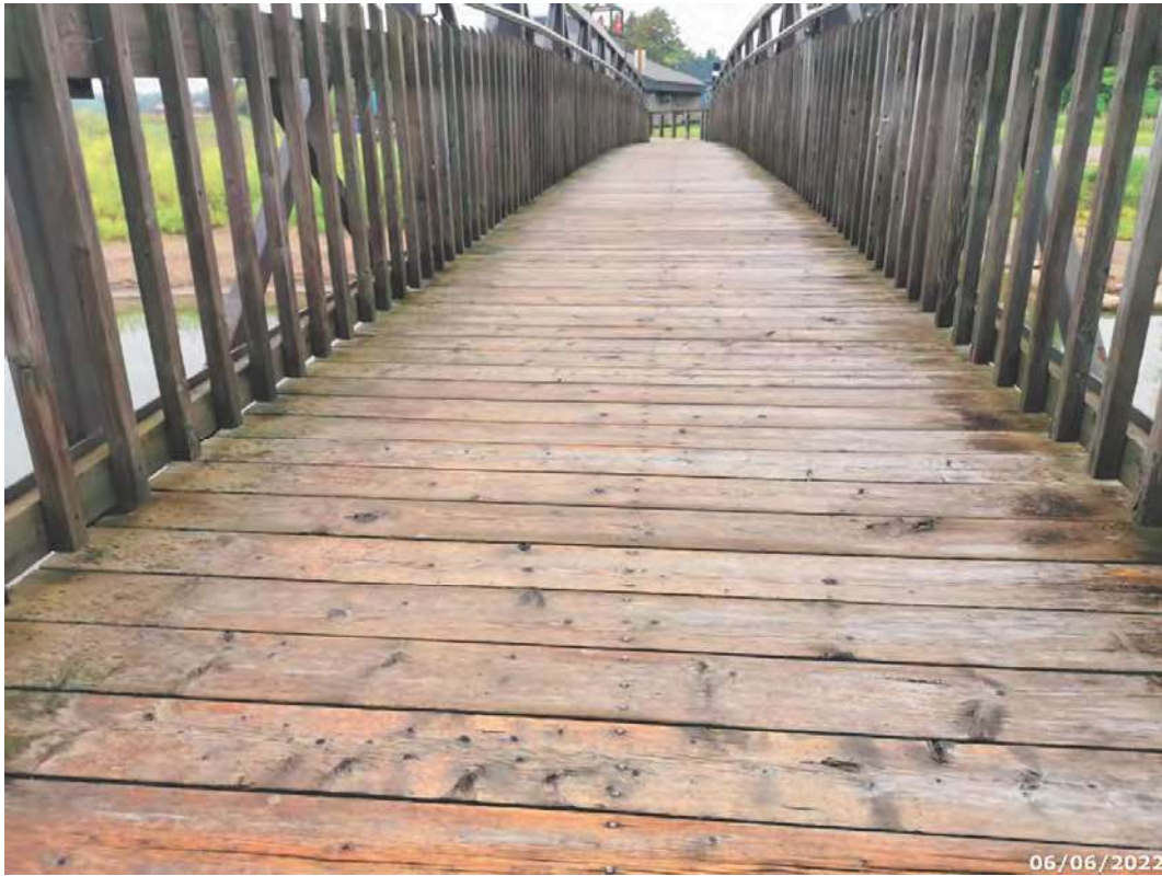
Typical deck wearing surface
