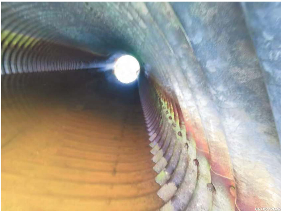
Looking South Along West Barrel Wall
