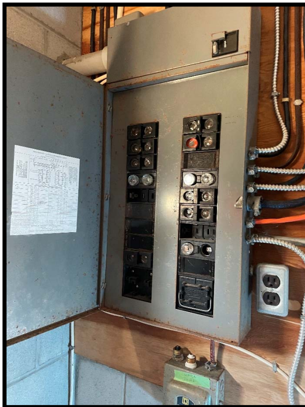
Photo 8 – Fused Electrical Panel
