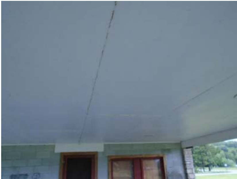
Photo 4: View of Pavillion Ceiling drywall – sample collected
