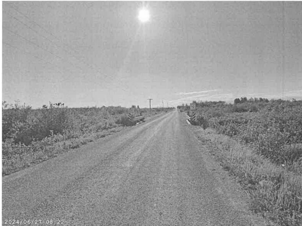
Looking East over structure
