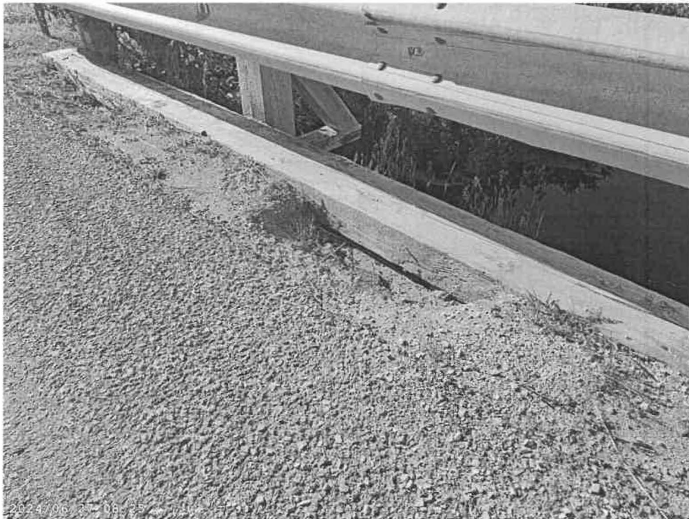
Curb and deck drain clear of gravel at scupper
