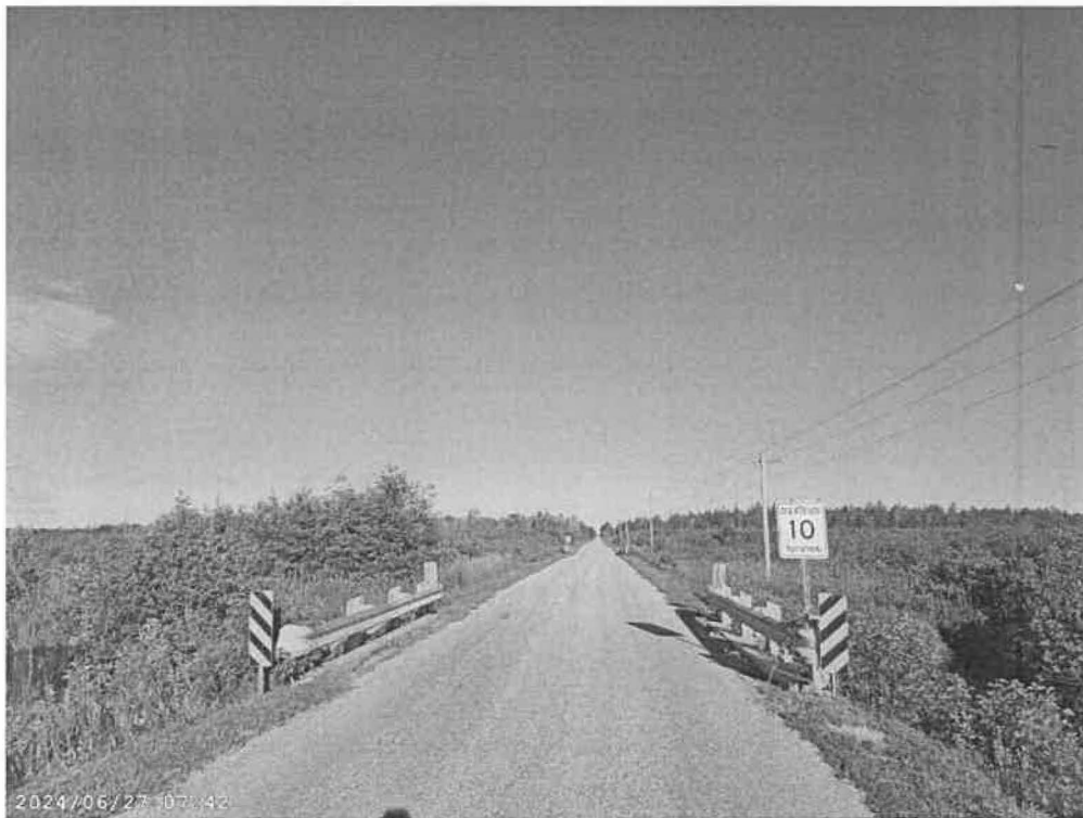
Looking West across structure
