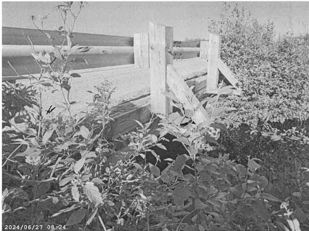
North elevation and railing support
