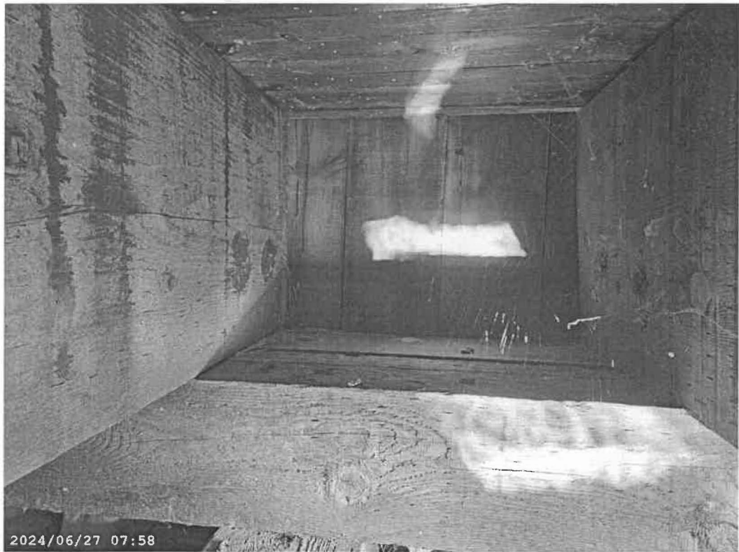
Interior bearing/ballast wall
