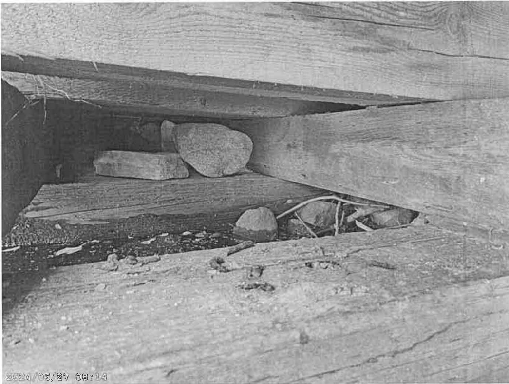
Loss of rock in crib
