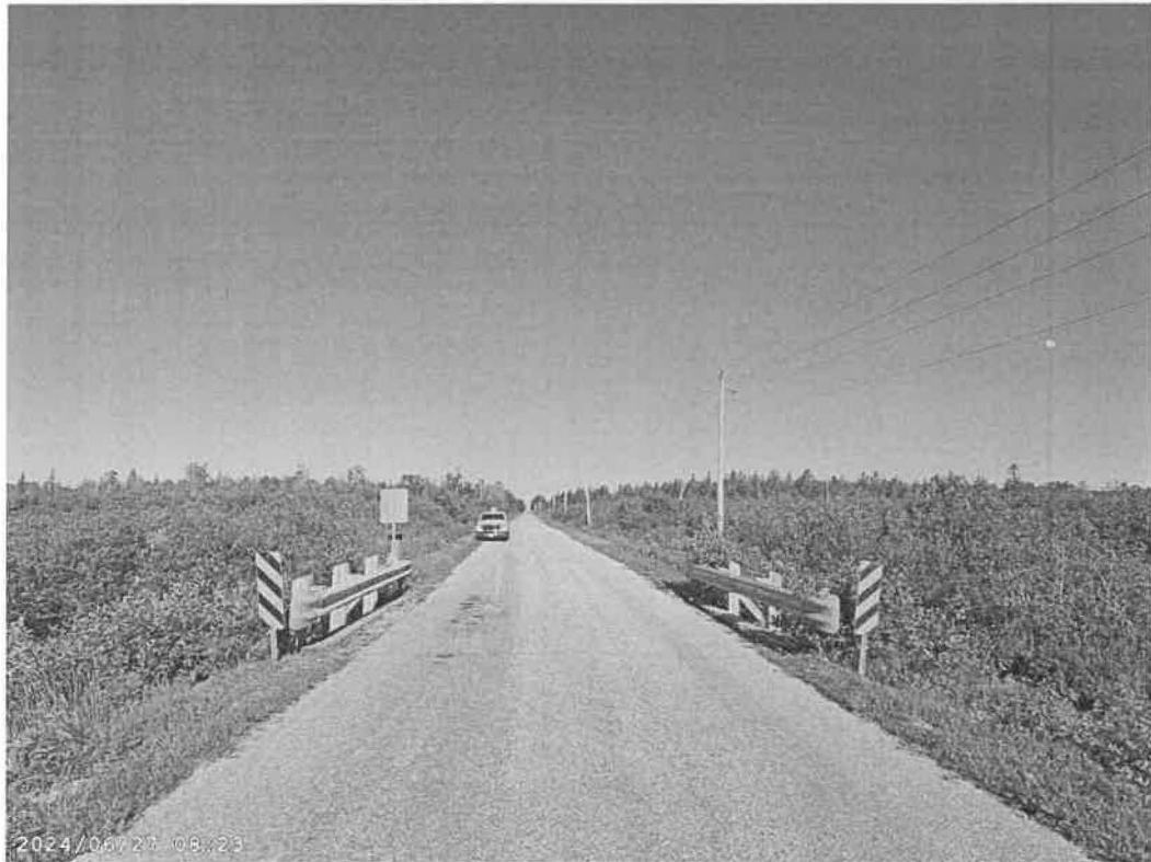
Looking West over structure
