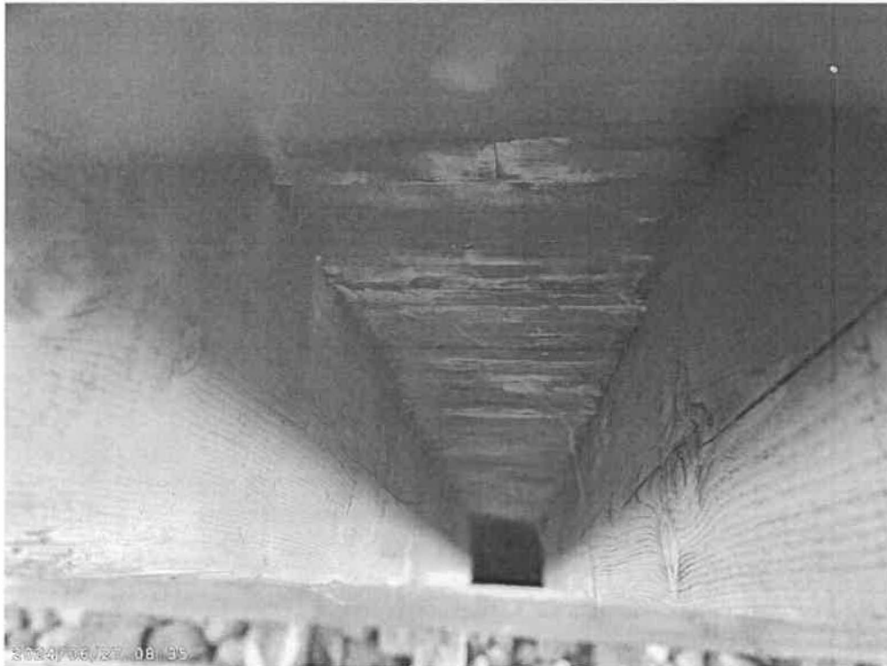
Interior deck soffit
