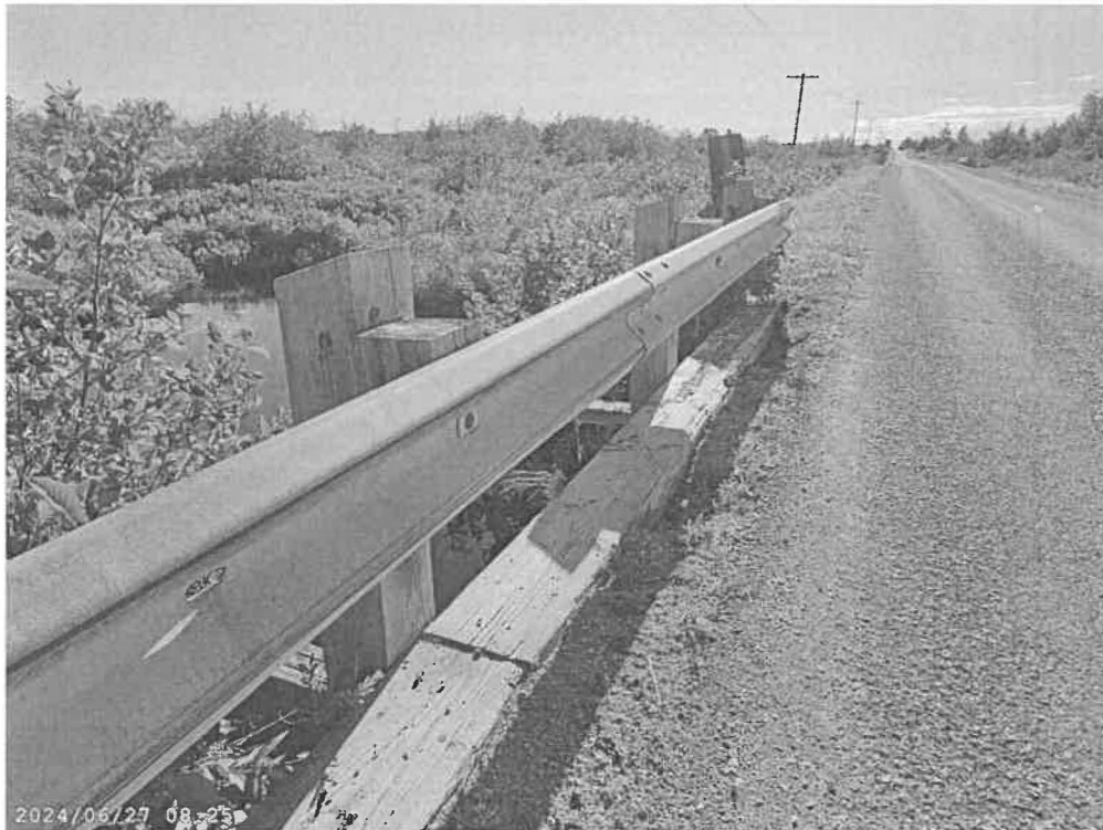
Typical curb and railing system
