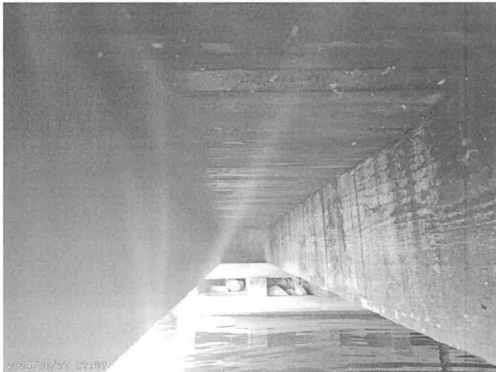
North exterior soffit
