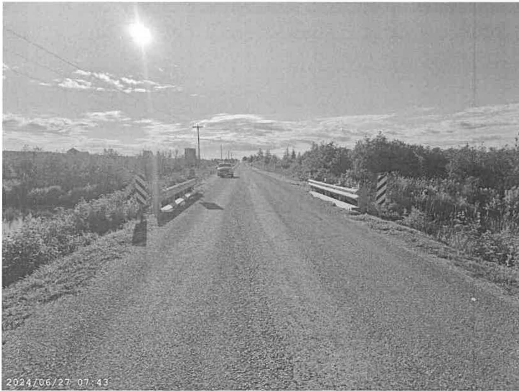
Looking East over structure
