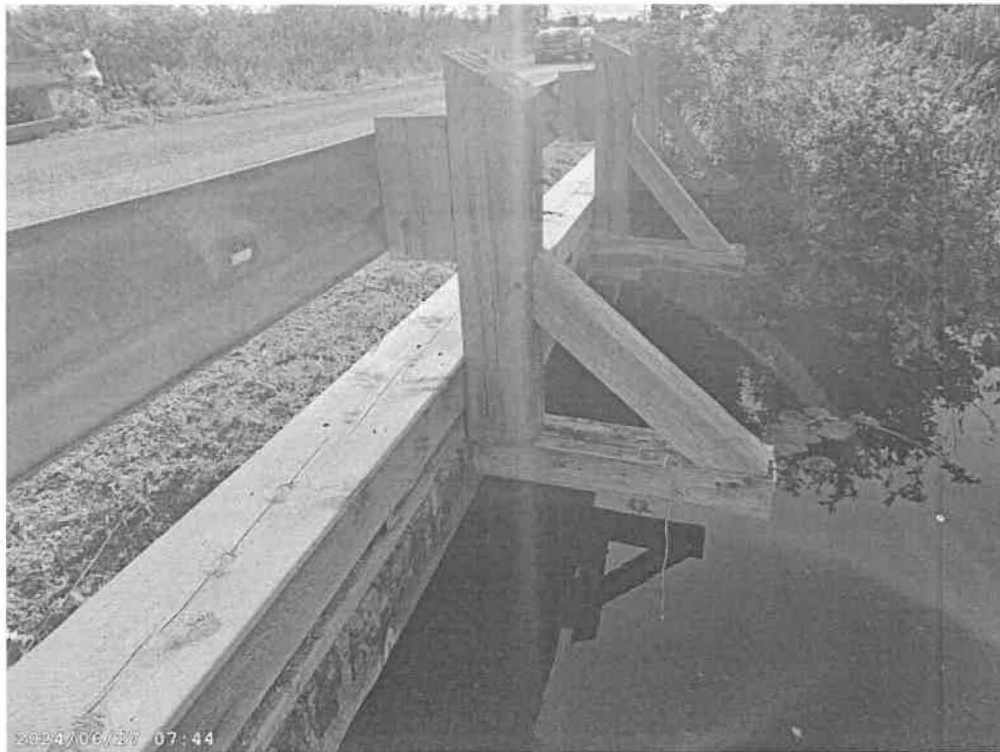
Typical railing posts and supports
