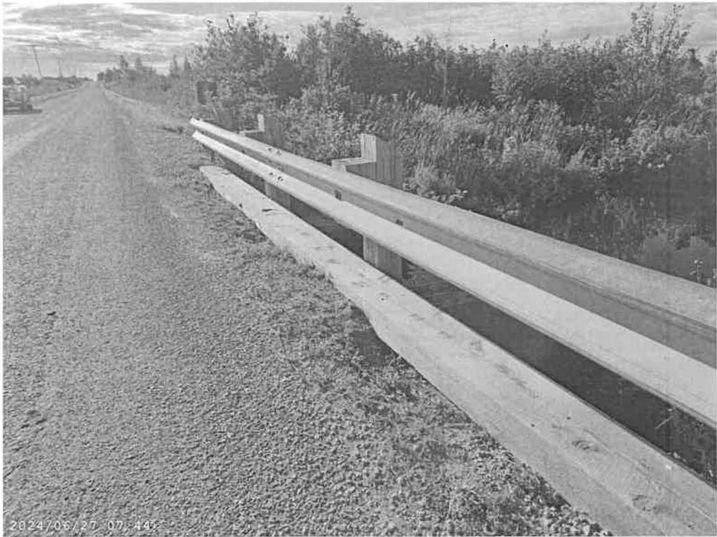
Typical curb and railing system
