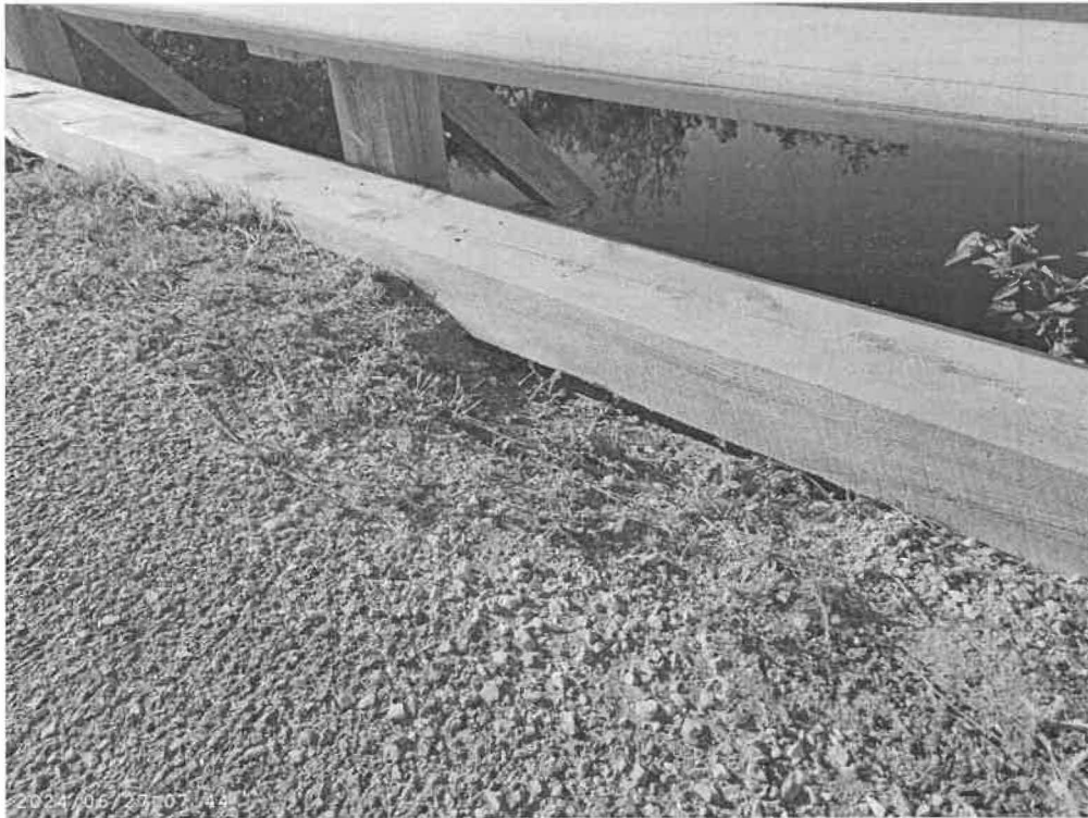
Deck drain to original scupper
