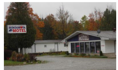
Commercial Fixed-roof Accommodation in Mindemoya in need of façade improvements
