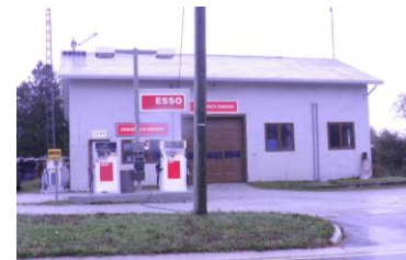
Potential Brownfield redevelopment opportunity: Garage for sale in Providence Bay
